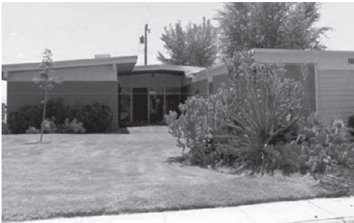
Older privatized housing at Holloman Air Force Base, New Mexico
