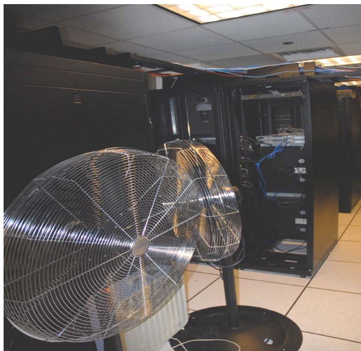
Figure 2. Fans Cooling Server Equipment
