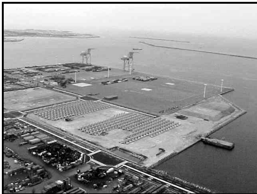
Figure 1: NPICT Aerial Photo
