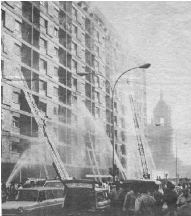
Fire scene from street as rescue operations became more consolidated. Note reach of USAF fire ladder, far right. (Photo from private collection of SMSgt Pighini, USAF, ret.)
