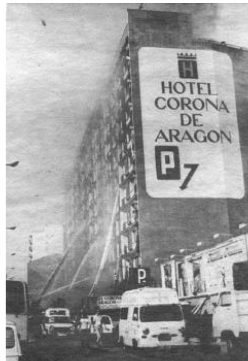
Fire scene from street. Note limited reach of ladders. (Photo from private collection of SMSgt Pighini, USAF, ret.)
