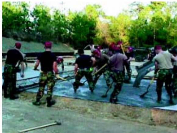
RED HORSE troops place approximately 30 cubic yards of concrete for the middle of three 6-inch pads for the covered range facility. (Photo by Capt Erik
