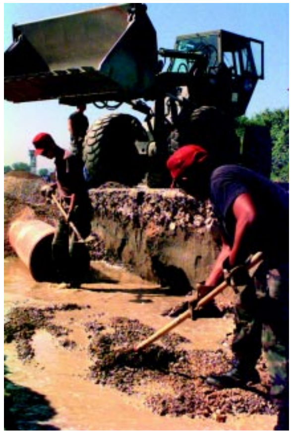
823rd RED HORSE Squadron personnel from Hurlburt Field, Fla., install drainage pipes along the main road leading to Rinas Airport near Tirana, Albania. (Photo by TSgt Cesare Rodriguez)
