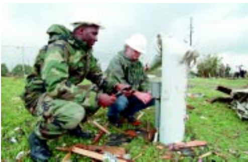
A1C Charles Chase and Carey Hill, both of the 72nd CES, isolate an electric pole that was blown down by the tornado at Tinker AFB, Okla. (Photo by Dave Faytinger)
