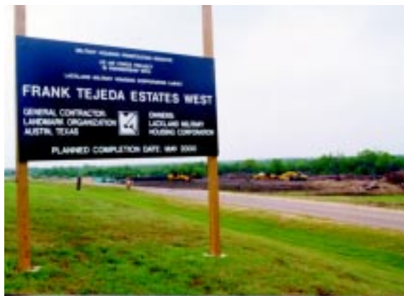
The developer broke ground on the construction site in April and is in the process of constructing the “model units” for the development. Completion of the first units is anticipated this fall with all units expected to be complete before the end of the year 2000. (Photo courtesy 37th Training Wing Public Affairs)
