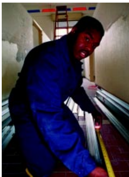
SSgt Shannon Fortune, 31st CES, Aviano AB, Italy, measures metal studs for the dormitory renovation. 31st CES craftsmen performed the majority of the work on the dormitory. (Photo by A1C Scott Nichols)
