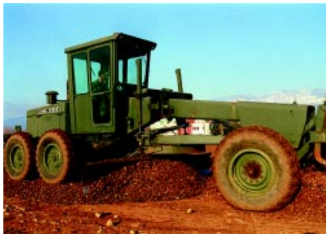
SSgt William Chilcott was part of the 31st CES team that accomplished a lot of beddown in a short time at Aviano AB, Italy. Here, earth is leveled and compacted in preparation for construction of Caserma Barbarisi, the tent city home for personnel supporting Operation Allied Force. (Photo by MSgt Raul Navas)
