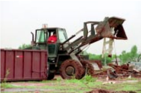
Chuck Littlejim, 72nd CEG, removes part of the fencing that used to surround the horse stables on Tinker AFB. The stable area was severely damaged by the May 3 tornado. (Photo by Margo Wright)
