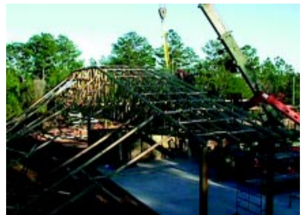
RED HORSE troops use a crane to lift into place one of the 96 truss sections and secure it to the horizontal beams. (Photo by MSgt Joseph Ondo)
