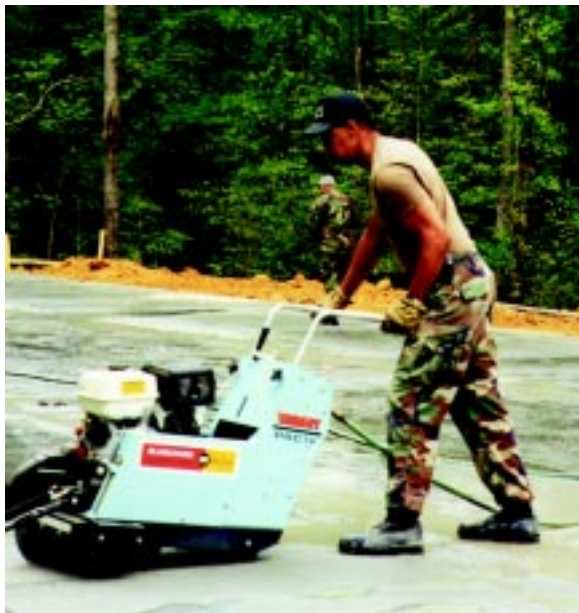
TSgt Bruce Thompson, 169th CES, saws joints in the concrete floor of the new education center at Congaree Swamp. The project was part of his annual training.
