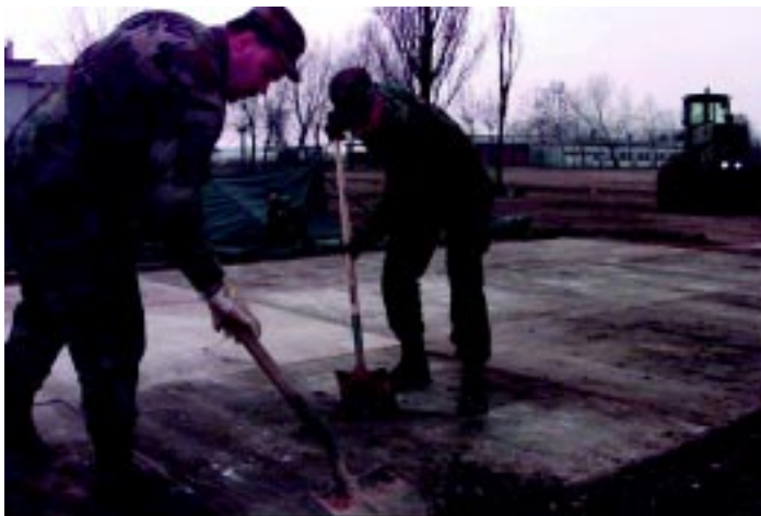
SSgt Angel Montalvo and TSgt Mark Kruse ( below ) and SSGts Al Johnson and Gardner Jones ( right ), from the 86th CEG at Ramstein AB, Germany, help construct the field kitchen at Aviano's tent city. (Photos by MSgt Keith Reed)
