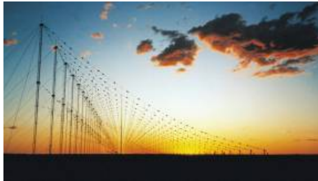
Figure 80. The JORN Transmission Antenna Array (From [108])
