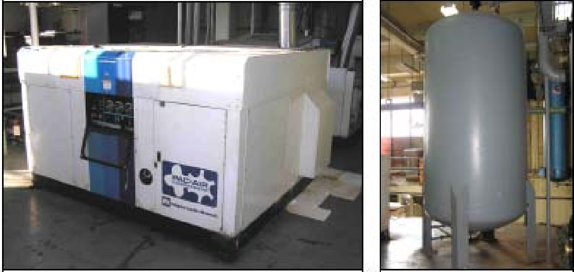
Figure 13. Photographs of one air compressor, and the receiver tank located in the compressor room (Helfrich, 2007:42)
