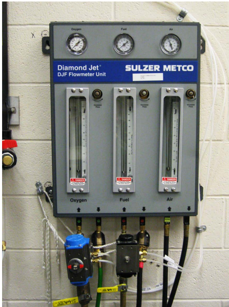
Figure 14. DJF Gas Flowmeter Unit
