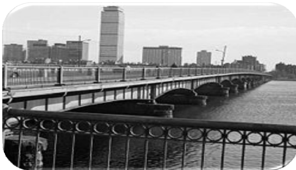
Figure 19. Massachusetts Avenue Bridge, Boston, MA, from [18]
