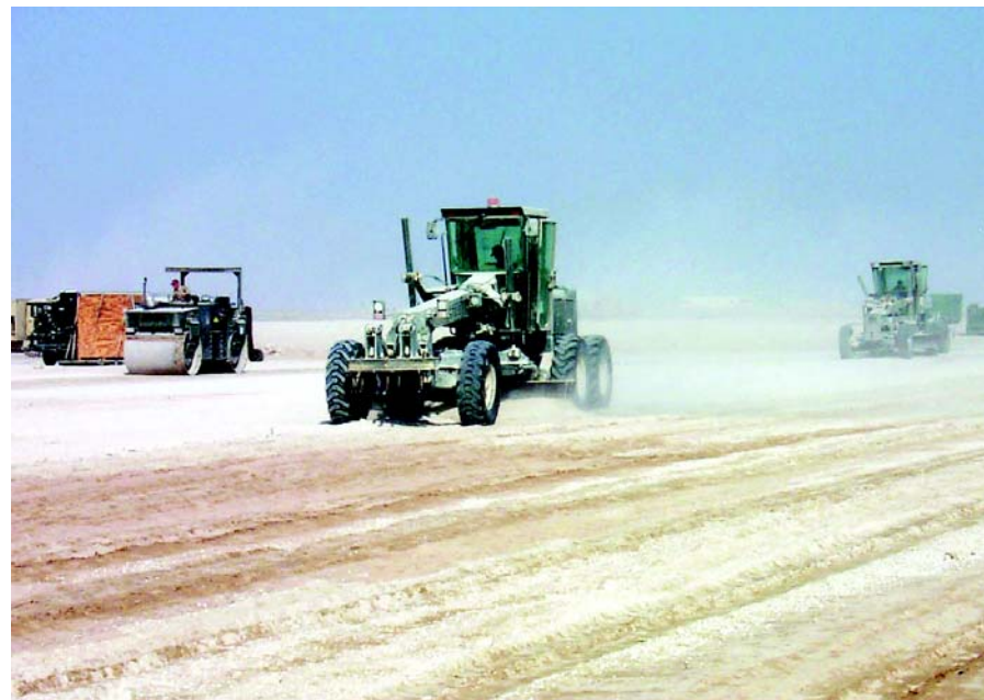
(From left) SSgts Tracy McBride and Jeramy Isaac and A1C Ryan O’Connell, all from the 823rd RHS, construct an equipment marshalling area for the air terminal operations center at a deployed location. (Photo by TSgt Carole Steele)
