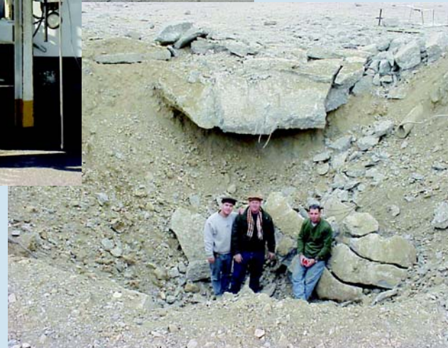
Bombs dropped from B-52s left craters on airfields like this one in Kabul that were more than 30 feet across and deep enough to hold several 823rd RED HORSE Squadron members.
