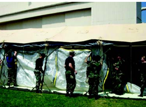
305th CES members practice setting up the new Transportable Collective Protection System, or TCPS. (Photo by Steven Robertson)
