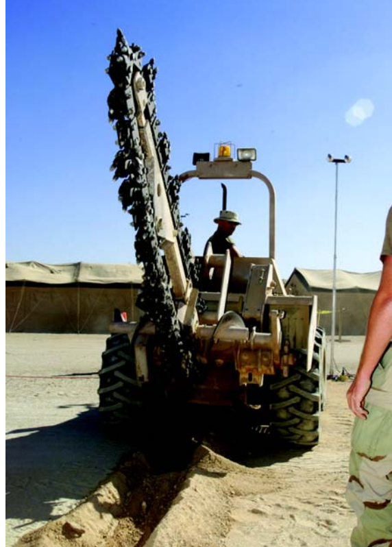
Digging a trench at a forward-deployed location Nov. 9. (Photo by TSgt Marlin Zimmerman)
