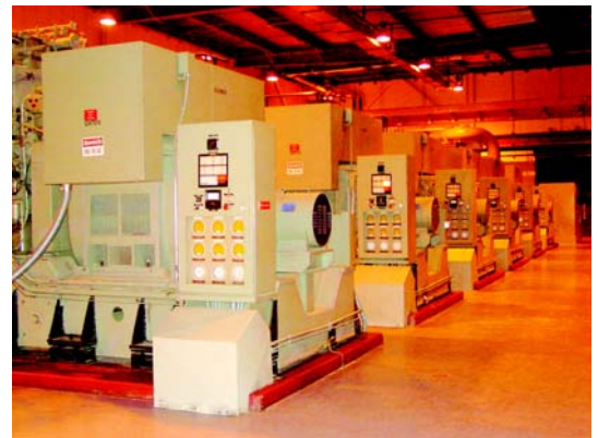
A total of seven diesel generators make up Schriever’s power plant and produce an astounding 15 megawatts of power.
