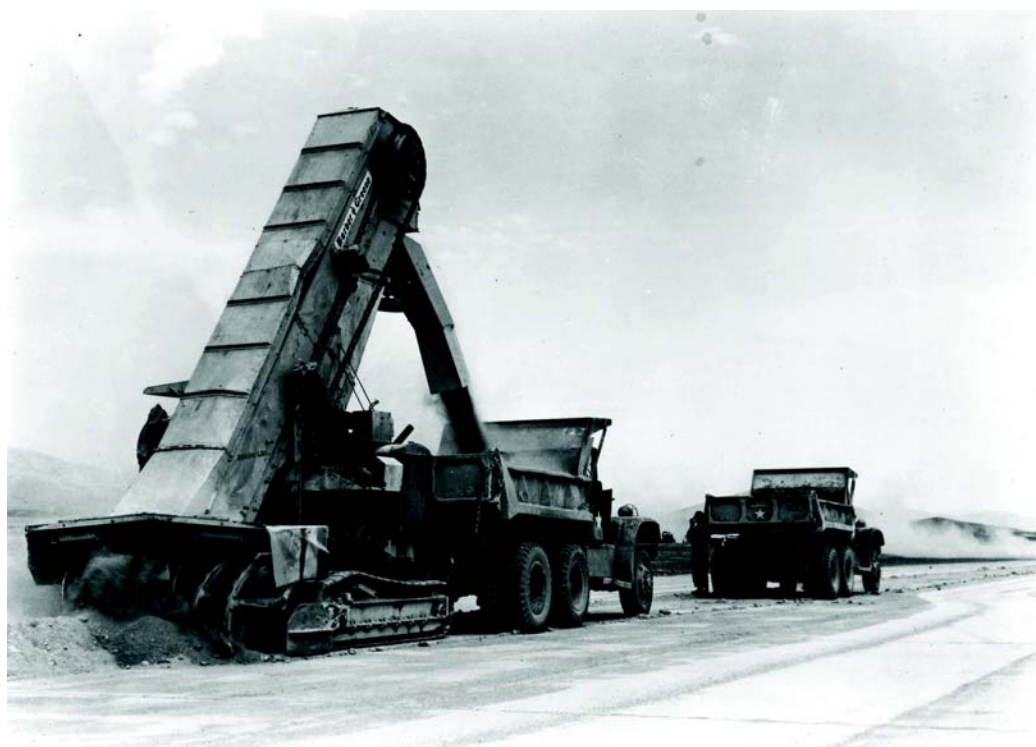
Trucks use a self-propelled conveyor loader to remove the curing sand from a 9,000-foot runway completed by the 930th EAG. (USAF photo)
