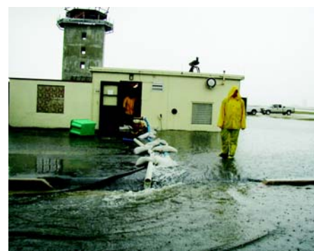
(From top to bottom) Approximately 3 feet of water stood in the basement of the West Airfield vault when the top photo was taken and 4 feet when the second photo was taken. David Washington (in doorway) and SrA Andrew Diehl, both from the 12th CES, at Randolph's West Airfield Vault. Approximately 30,000 gallons was pumped out of the basement that day. (Photos by MSgt Luis A. Adams)
