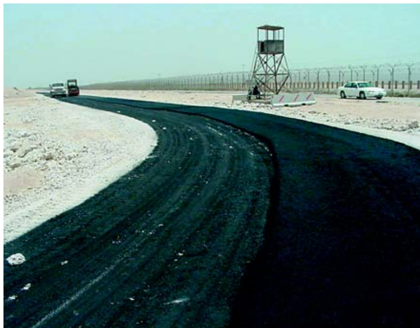
Crosser Boulevard was constructed to redirect vehicle search area traffic at Camp Snoopy, Qatar. RED HORSE units completed construction despite 120-degree temperatures. (Photos courtesy 200th/201st RED HORSE)
