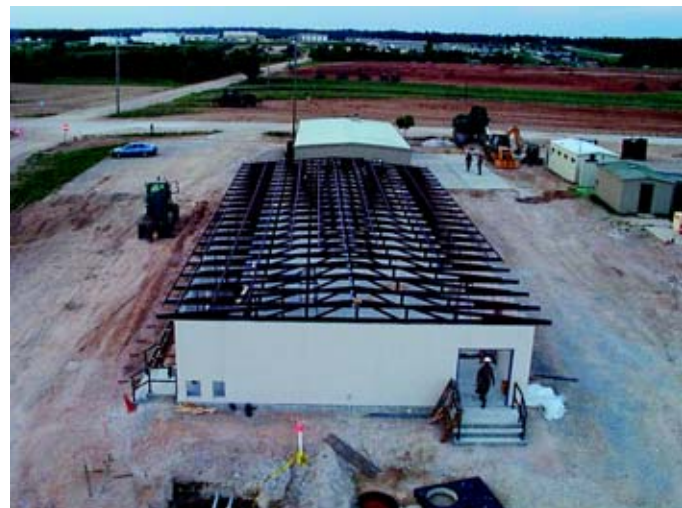
(Top) Construction of an observation tower for monitoring heavy equipment training. (Above) The new classroom facility under construction by the 820th RHS. (Photos by MSgt Ken Willard)
