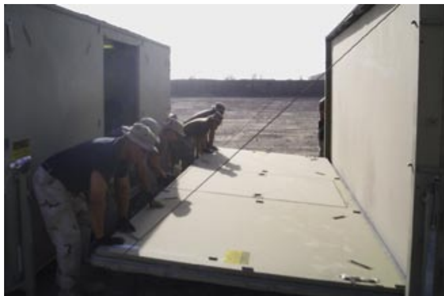
A team lowers the floor panel and vertical wall that supports the roof and ties the side walls. (photo by SrA Dora Sherrill)
