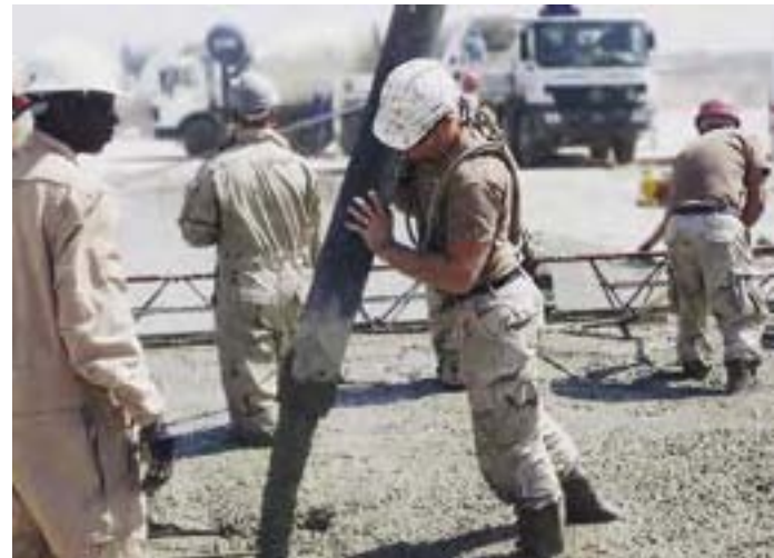
SrA Terrell Jackson (left) and SrA Andrew Hikes, 557th ERHS, direct a high-reach concrete pump during the heliport construction project in Southwest Asia. (U.S. Air Force photo)
