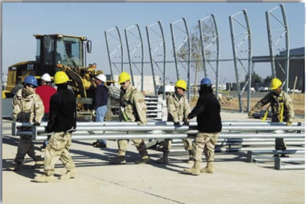
Airmen from the structures shop of the 332nd ECES position an arch during construction of a shelter for Hunter unmanned aerial vehicles at Balad AB, Iraq. (photo by A1C Chad M. Kellum)
