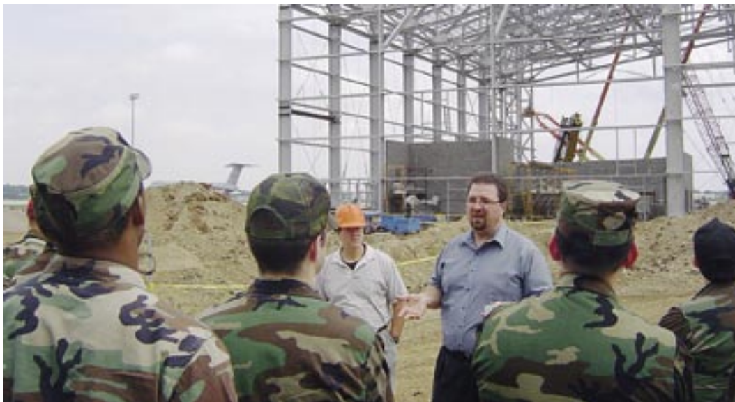
ENG 481 students observe hangar construction techniques as part of their coursework. (photo by Capt Brian Ballweg)
