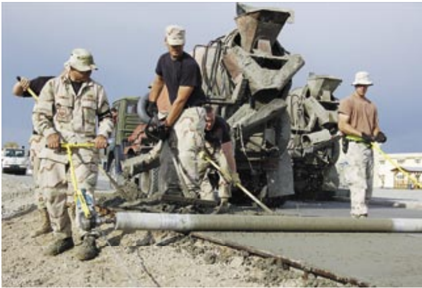
Members of the 376th ECES “Dirt Boyz,” SSgt Jeffrey Trombley (left) and TSgt Bryce VanOverbeke screed freshly placed concrete on a sidewalk, while SSgt Adam Ruter (center) rakes the concrete level. SSgts Trombley and Ruter are deployed from Grand Forks AFB, N.D., and TSgt VanOverbeke is deployed from Elmendorf AFB, Alaska. (photo by the author)
