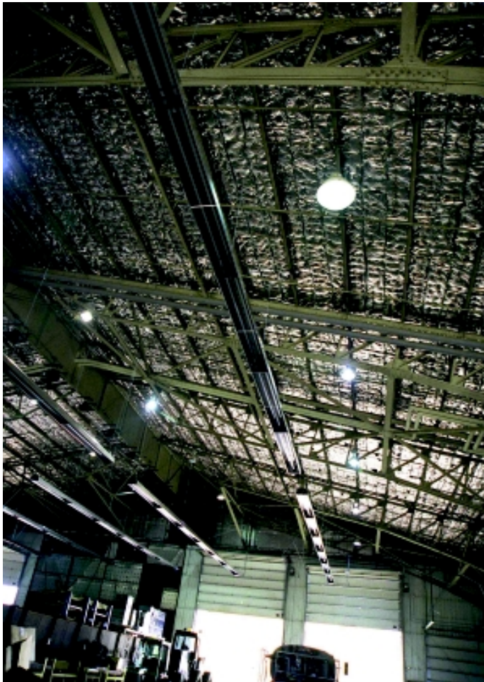
Grand Forks AFB used an ESPC contract to fund base infrastructure improvements such as these gas-fired, infrared heaters. (Photo by TSgt Charles Morris)
