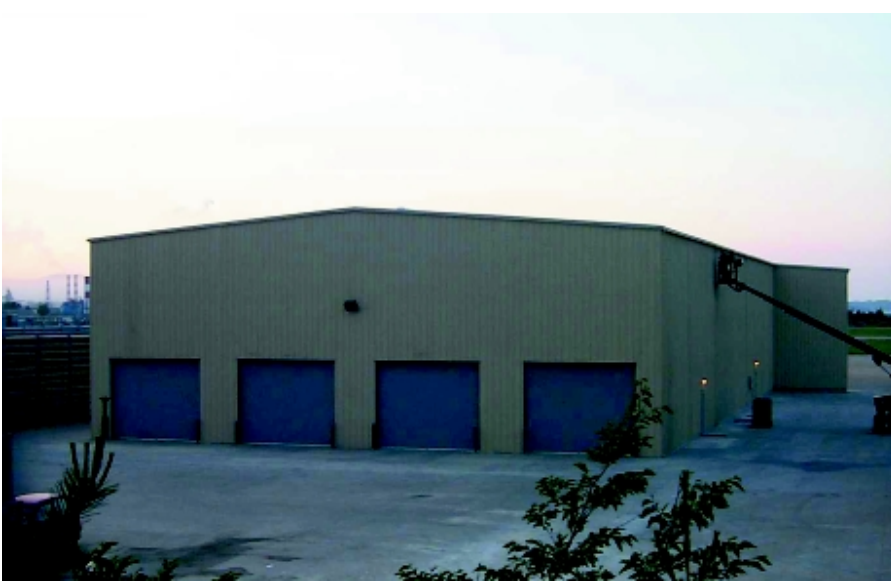
(Top) The front of the 8,000 square foot hangar accommodates an 80 foot by 28 foot hangar door to enable USMC helicopters to be moved into and out of the facility. (Above) The rear of the hangar is for storage of materiel handling equipment with access through four roll-up doors.
