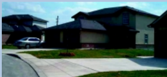
More than 420 new homes for enlisted service members E-3 to E-7 are nearing completion at Lackland AFB. This was DoD's first housing privatization project. (DoD photo by Linda Kozaryn)
