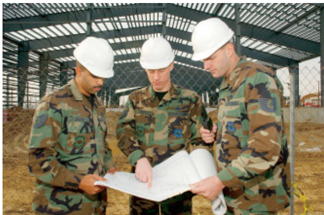
TSgt Jose Dicupe, HVAC NCOIC; TSgt Bradley Warren, Facility Maintenance NCOIC; and MSgt Christopher May, Superintendent of Facility Maintenance Element (photo by Carlos Cintron)
