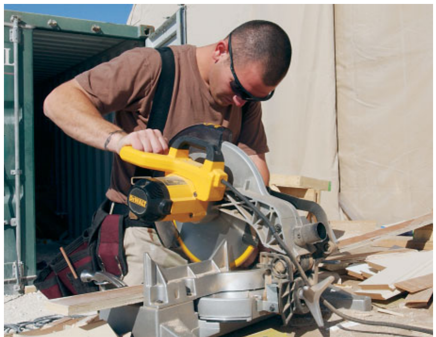
A1C Dan Thompson trimmed molding at the CAOC.
