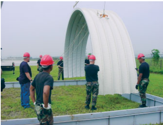
PACAF structures troops learn how to erect K-span facilities during vendor training at Osan AB, Republic of Korea.
