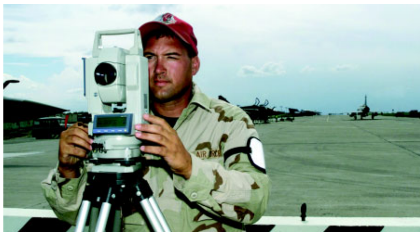
SSgt Phillip Boss, 200th/201st ERHS engineering assistant, uses a theodolite to measure the vertical and horizontal angles of a new taxiway extension in Kyrgyzstan. (Photo by MSgt Jerry King)
