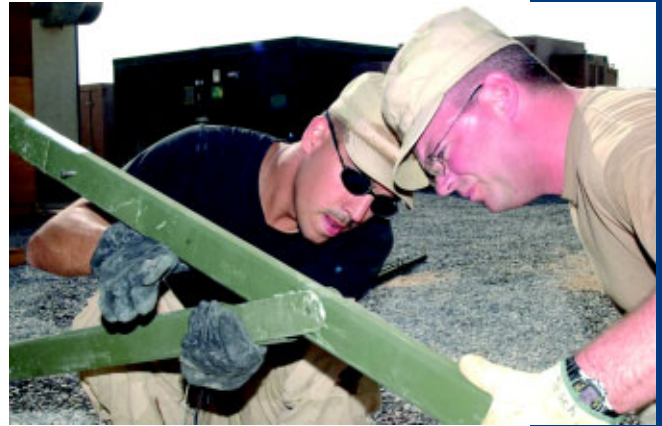
SrA David Dottavio (left) and TSgt Gregory Tesch, both of the 320th ECES, put a tent frame together as they prepare to extend the base dining facility Feb. 21.
