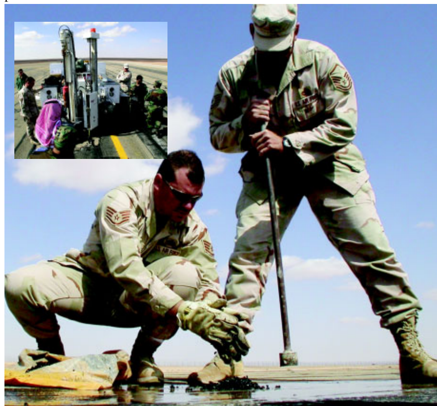
(Above and inset) MSgt Scott Melton and SSgt Greg Welch patch a core hole on an airfield as interested locals observe. Everywhere the team went, the local populace was curious about their work.
