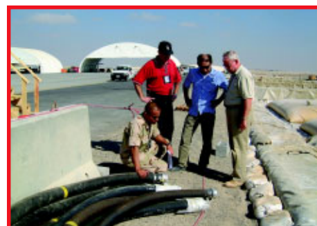
(Top to bottom) The 380th ECES broke ground Christmas Day 2002, excavating and grading land for a new fuel farm at their forward deployed location. Local contractors perform quality control checks on the piping system. Capt Juan Alvarez, 380th ECES Engineering Flight chief, and construction manager Ken Lombard of RMS worked with contractors to complete the project, which resulted in a wartime throughput averaging over 2 million gallons of jet fuel per day. (Photos courtesy 380th ECES)
