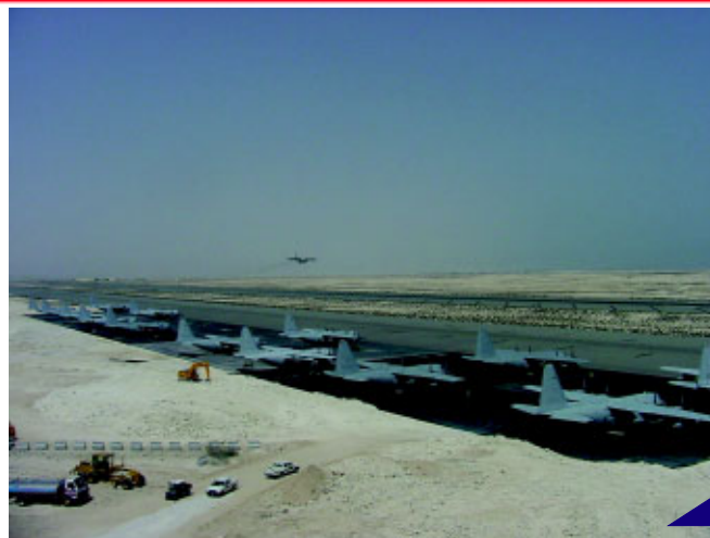
The SWA Delivery Team resolves planning, programming and construction issues for civil engineers in forward operating locations to expedite projects such as this aircraft parking ramp built by a Prime BEEF team for Operation IRAQI FREEDOM, and beddowns such as the tent city at Manas, Kyrgyzstan, below. (Tent city photo by CMSgt Andrew Stanley)
