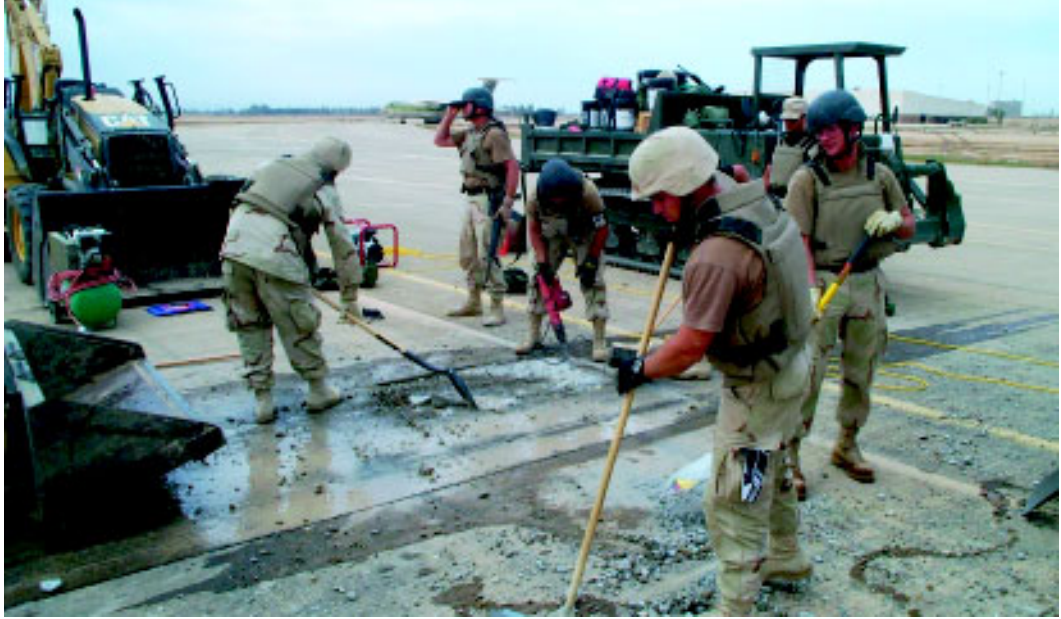
An ARH team repairs a spill on a runway at an Iraqi air base using equipment from the MARES: CAT 420 backhoe (left) and IHI IC-45 crawler carrier (right).
