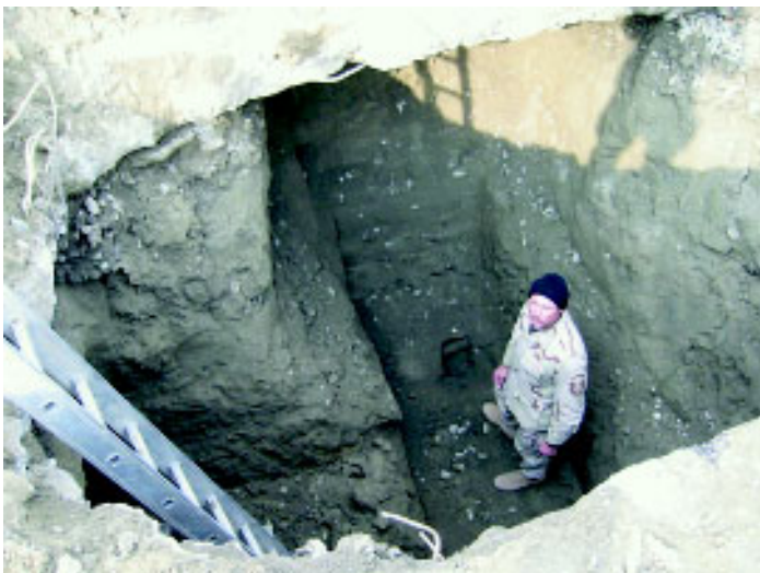
MSgt James E. Brewster, 379th ECES, stands at bottom of hole excavated to find the entry route of UXO located beneath runway in Afghanistan. (U.S. Air Force photo)
