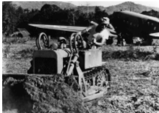
Left: A crew loads engineering equipment into a Douglas C-47 of the 1st Air Commando Force at Tamu, Burma. Right: An airborne engineer uses a miniature bulldozer to lengthen a runway at Tamu, Burma. Below: Glider-landed aviation engineers tow their glider off the airstrip at Myitkyina, Burma. (U.S. Air Force photos)
