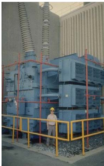
Figure 5-20: High-Voltage Power Transformer in New Jersey, USA, Before and After the Geomagnetic Super Storm (first and second image) on the 13th March 1989 and the Transformer Windings were Permanently Damaged in New Jersey, USA, During the March 1989 Geomagnetic Storm. Third image: destroyed transformer in South Africa in October 2003.
