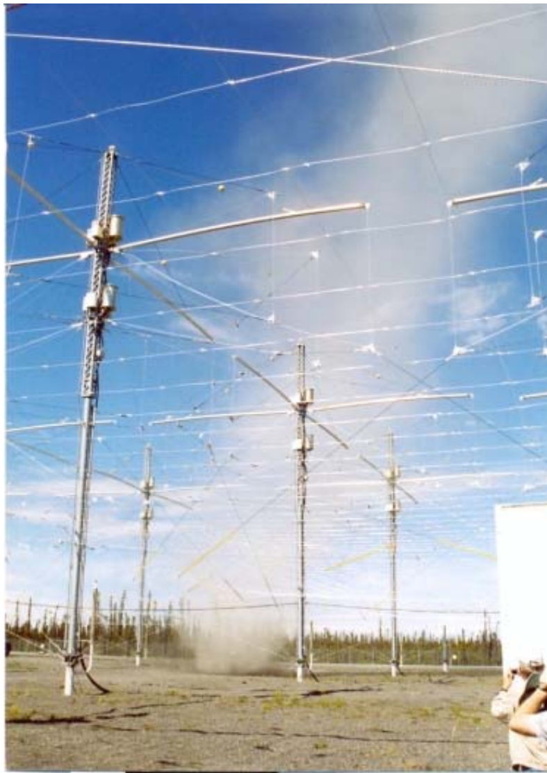
Figure 5-24: A High Power Antenna Field in Alaska (with a 'Dust Devil' in Background (image: F. Jansen)).
