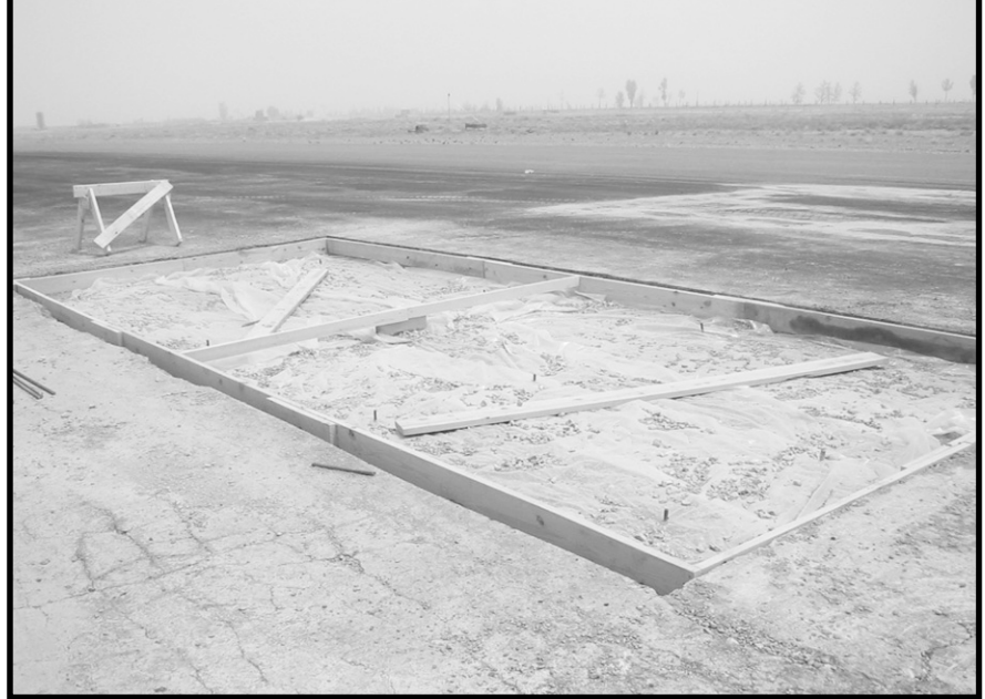
Offset framework, complete with vapor barrier, is ready for the arrival of the concrete truck and crew.
