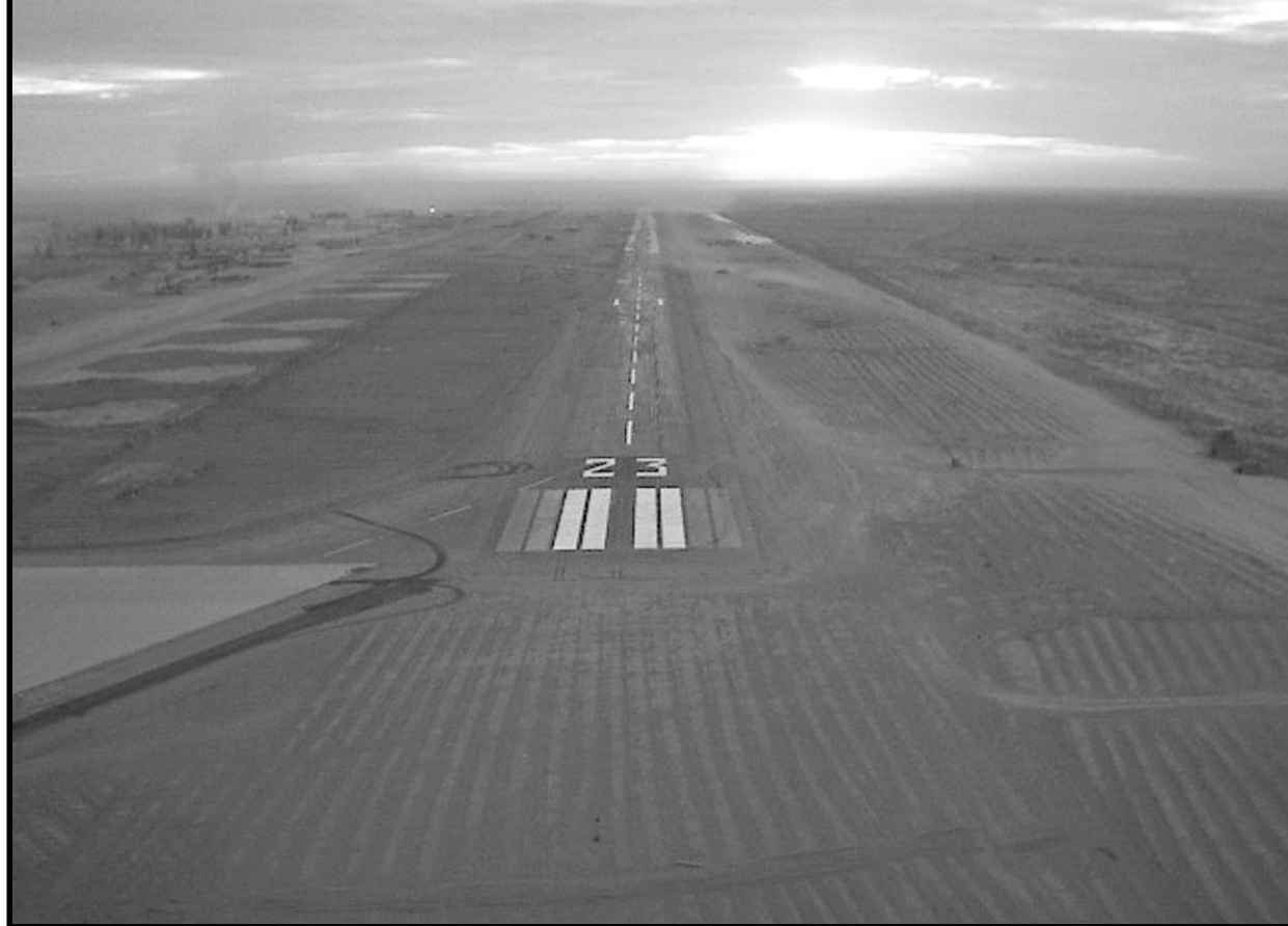
An overhead view of Runway 23 shows that Federal Aviation Administration-approved reflective paint, plus a recent application of asphalt sealant, can make a runway look new despite its age.
