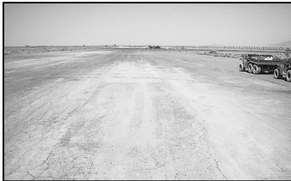
A recently stabilized soil patch is prepared for an application of dust control agent.
