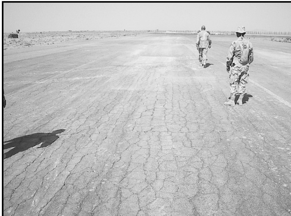
Task force engineers inspect a damaged section of asphalt.
