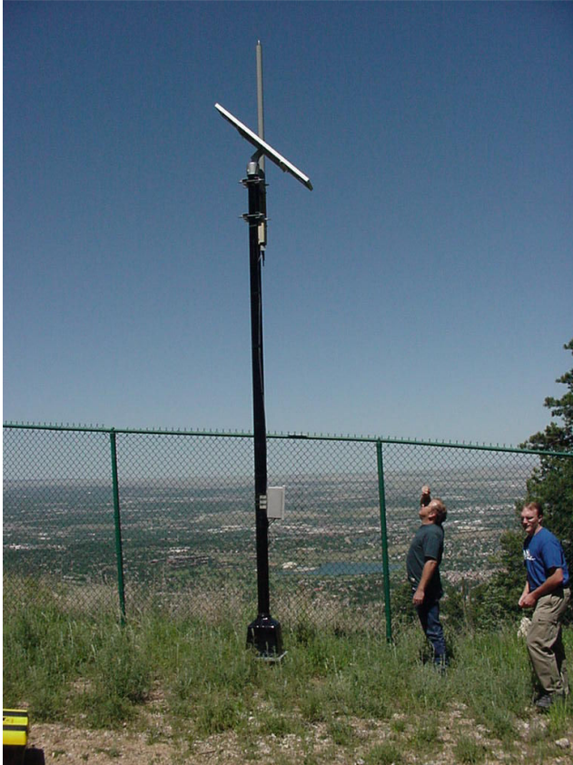
FIGURE 10 Stand-alone repeater antenna system overlooking Colorado Springs from the Air Force Academy.
