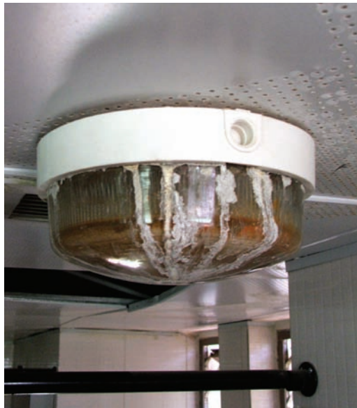
Site Photo 21. Urine-filled ceiling light.
