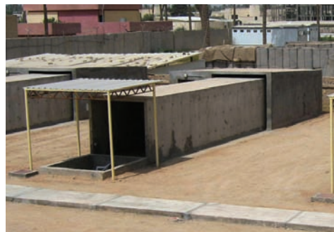
Site Photo 16. Pistol-firing station showing shooter's pit, firing tube, and target enclosure.
