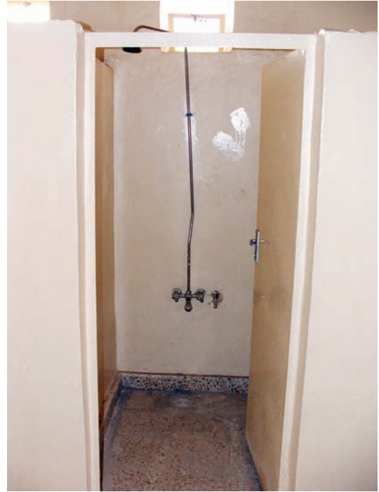
Site Photo 14. Shower facilities at the 2nd Brigade garrison showing a thin wall metal tubing shower fixture connected to the wall with a single screw clamp.
