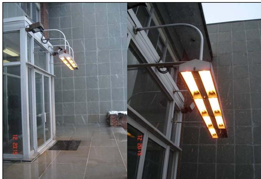
Figure 39. Infrared heaters above CRREL entrance.
