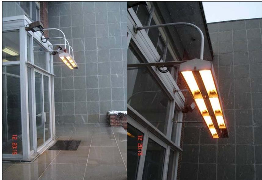
Figure 39. Infrared heaters above CRREL entrance.
