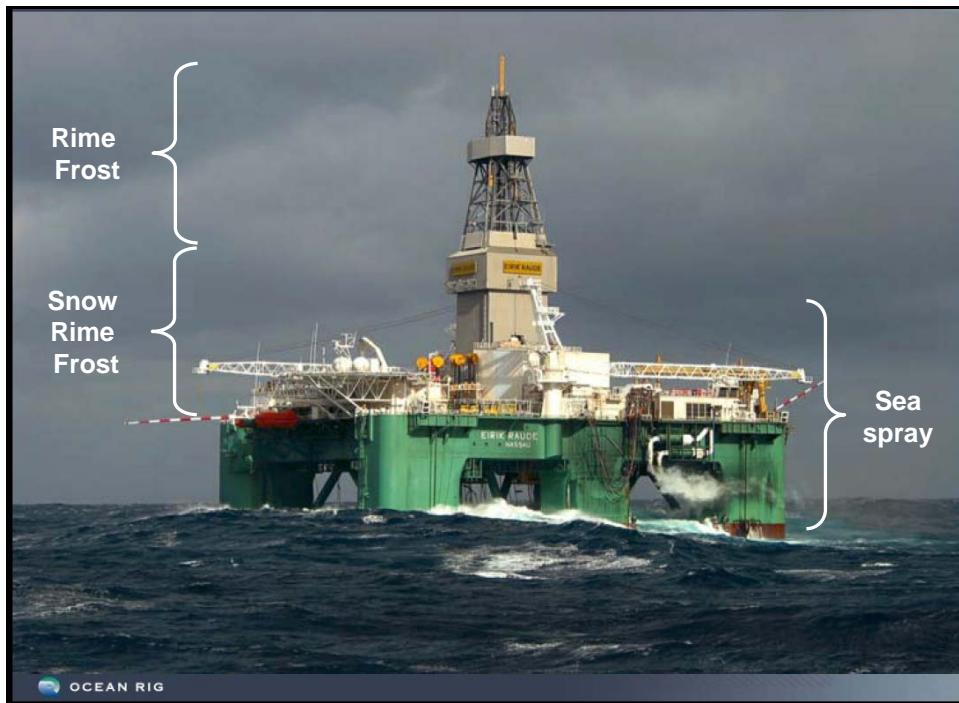
Figure 5. General locations where atmospheric icing (frost, snow, rime, and glaze) and superstructure ice (sea spray icing) would be expected to occur on a drilling platform such as the *Eric Raudé*.
