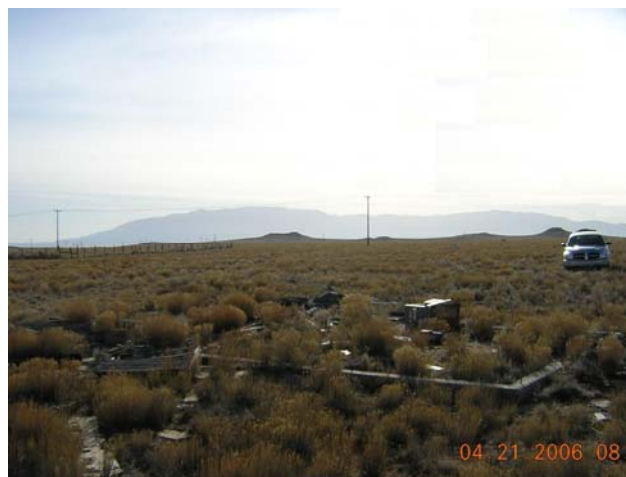
Figure 5-30. Ground reconnaissance of KPBR-AOI-3 found the remains of a building foundation and associated building debris. The area surrounding the foundation appears to have been excavated, which accounts for the depression.
