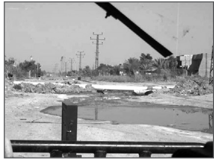
Figure 19. Typical Electric Grid infrastructure in Baghdad
