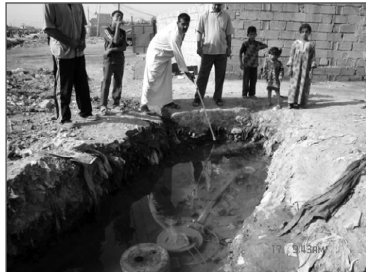
Figure 24. U.S. and Iraqi forces ongoing repair of major sewer and water point breaks in Sha'ab/Ur districts of Baghdad
