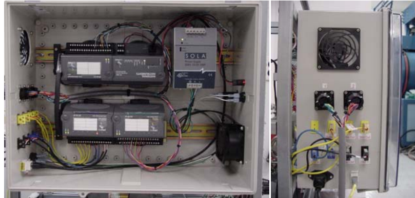
Figure 8: Control System Input / Output Modules
