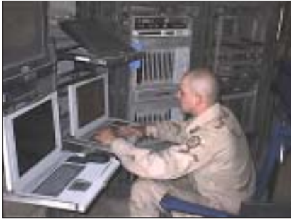
The 63 rd set up a technical control facility. Company B soldiers built a room in an old Iraqi building and turned it into the Tallil Air Base TCF.
