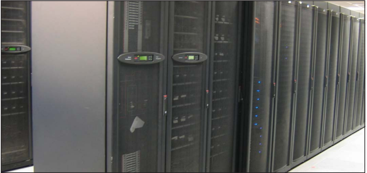
The datacenter above was built with scalability to support future customers, their missions, and allow multiple services to capitalize on a shared infrastructure. Air Force and Army systems located in this facility have proven the concept of a Real-Time Infrastructure can be successful.
