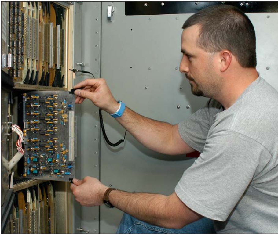
Brian Wesolowski installs a circuit card in an AN/TPS-75 Radar System shelter signal processor rack. Replacing circuit cards is part of the overhaul process for the radar system. Depot personnel have decreased the radar's overhaul time by almost 50 percent. Wesolowski is an electronics worker in Tobyhanna Army Depot's Surveillance Systems Directorate.
