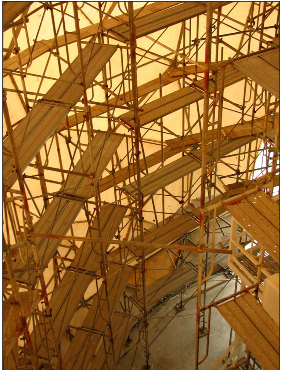
Scaffeling for maintenance of the interior of the 333rd Signal Company’s RADOME reaches the top of the 50-foot structure.
