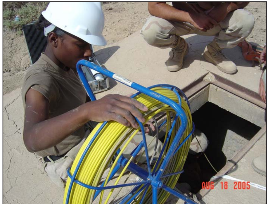
54th Signal Battalion Soldiers install fiber optic cable in Iraq.
