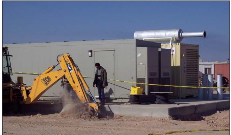
A worker watches the digging for the grounding ring outside one of the four 30-ft transportable shelters that make up the Tech Control Facility at COB Speicher.
