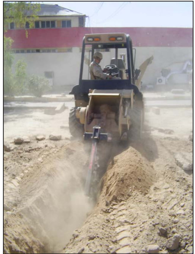
A ditchwrench installing communications infrastructure in Iraq.
