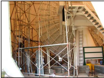
Scaffolding is prepared for interior maintenance of the 333rd Signal Company's RADOME.
