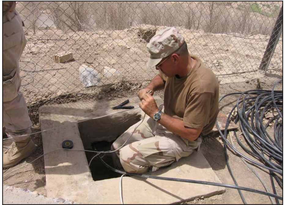
Soldiers of the 54th Signal Battalion install communications at Camp Victory in 2005.
