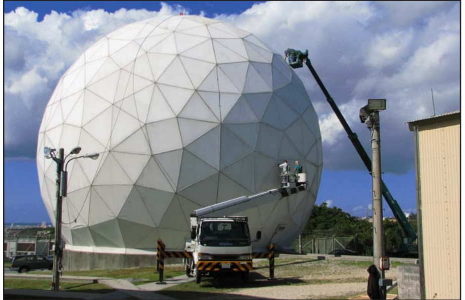
Tobyhanna Army Depot personnel refurbish the exterior of the 333rd Signal Company's RADOME.
