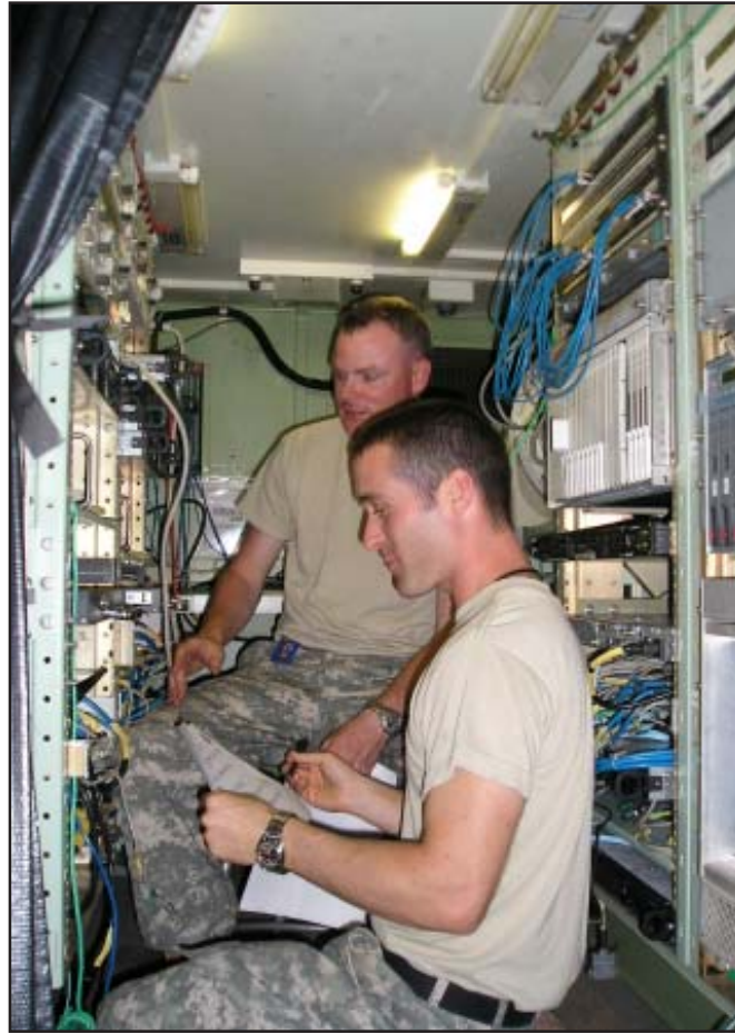
SSG Robert Martin (background) instructs SGT Malcolm Davis on the signal flow of the C4 team's base band node shelter.
