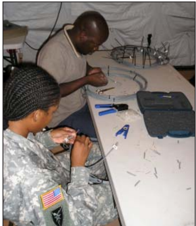
SGT Nicolette Jones and Lee Hatten terminate Category 5 cabling for use with an Air Force phone voice switch.
