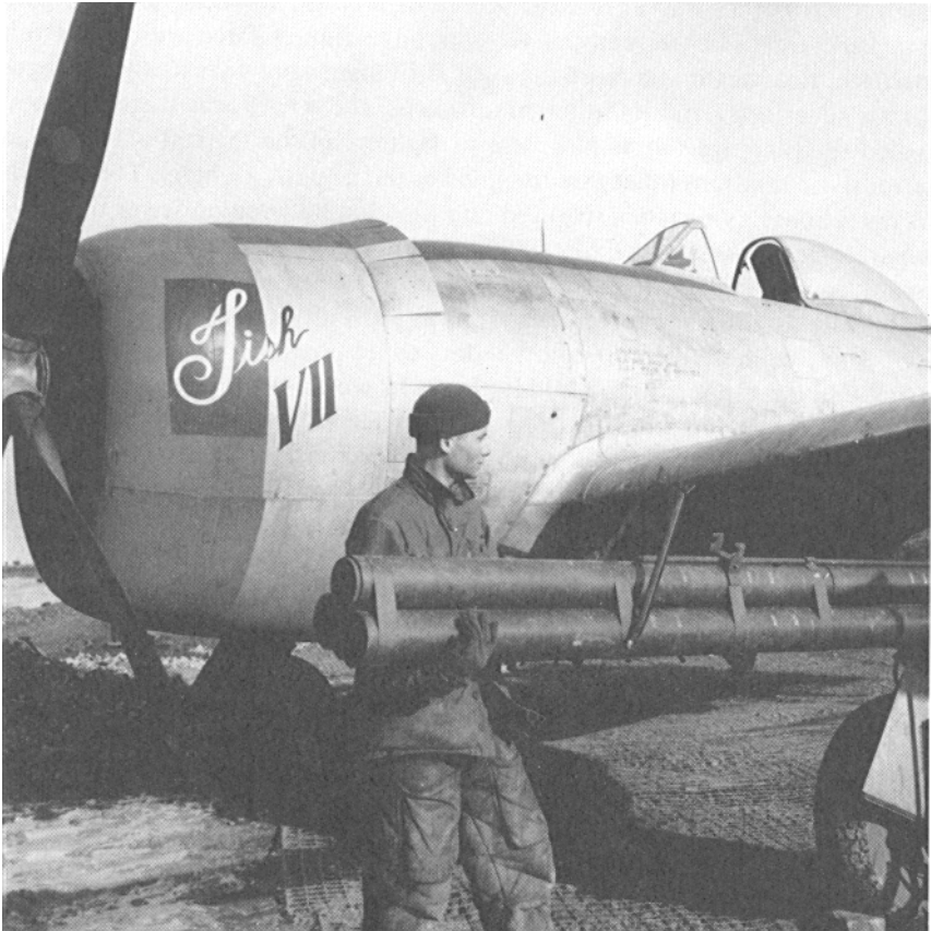
Ground crewman mounts a field-expedient rocket launcher on the wing of a P-47J Thunderbolt.
