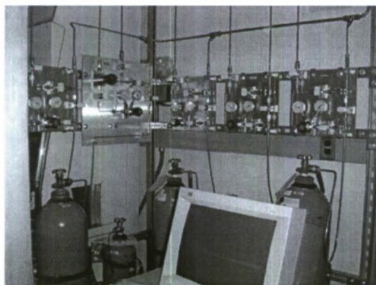
Figure 2) The inert gas panels for the ICP RIE system. The monitor in front is for a Rapid Thermal Processor.
