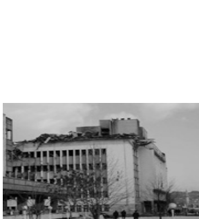
Telecommunication building in Prishtina
