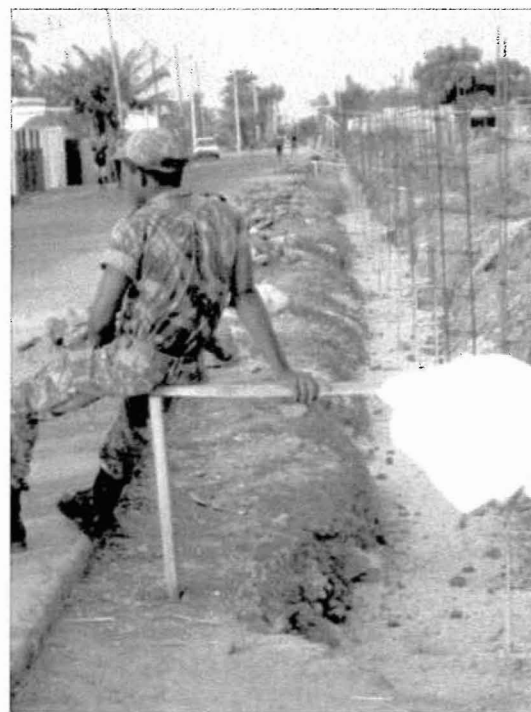
PHOTO: BRIDGETTE RICHARDSON Figure 6: Construction of a perimeter fence at the International Airport. Military personnel constructing security fence along the north perimeter. The villages (to the left) will be cutoff from their direct route crossing the runway.
