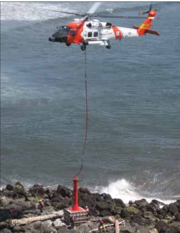
Coast Guard personnel install an aid-to-navigation to enhance marine safety along the Washington State coast.
