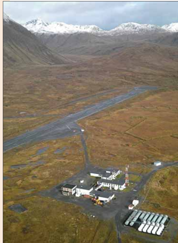
Coast Guard LORAN Station Attu as seen from the top of the antenna. The station is home to 20 Coast Guardsmen, the island’s only human inhabitants.
