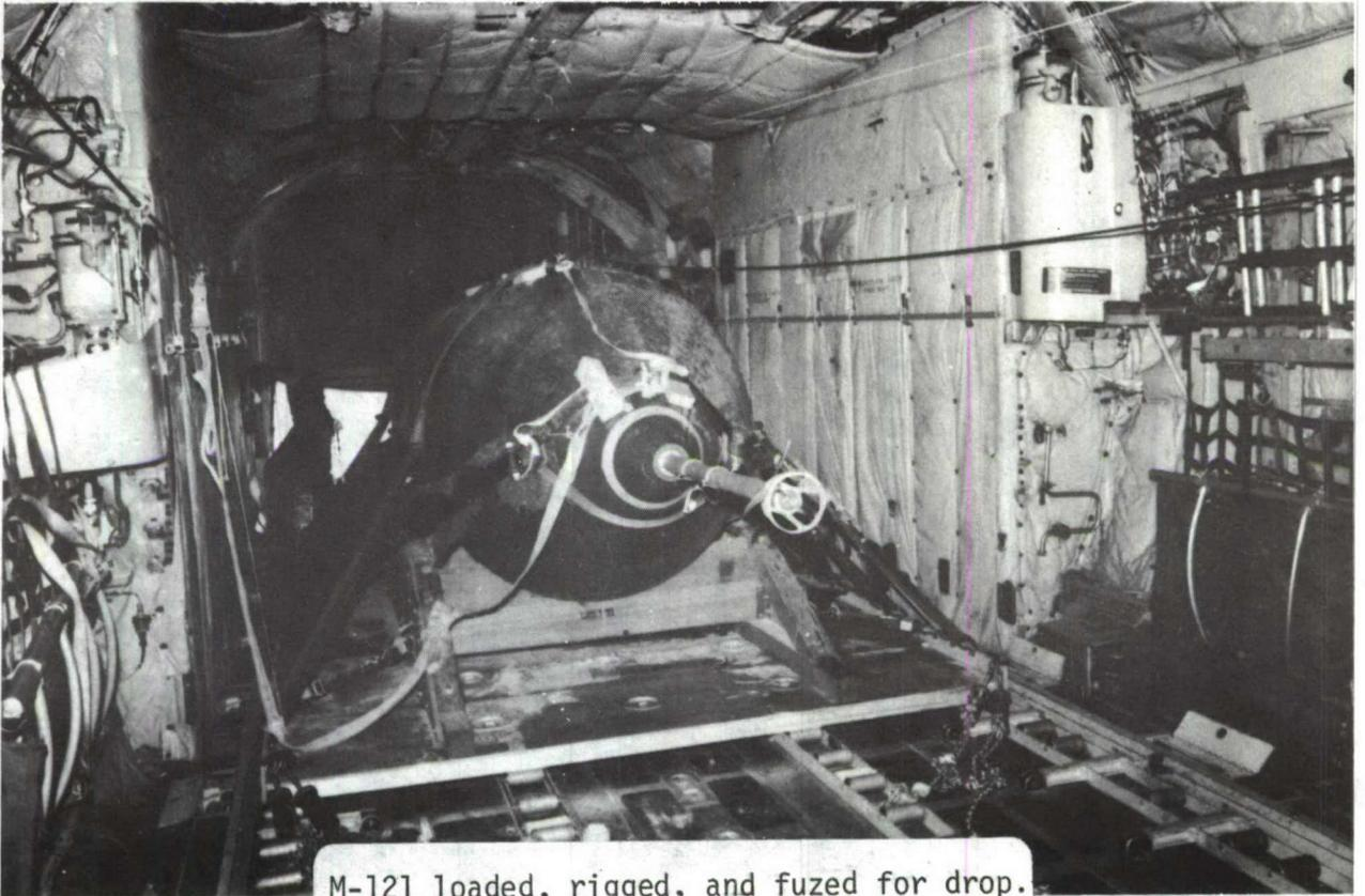
M-121 loaded, rigged, and fuzed for drop.
