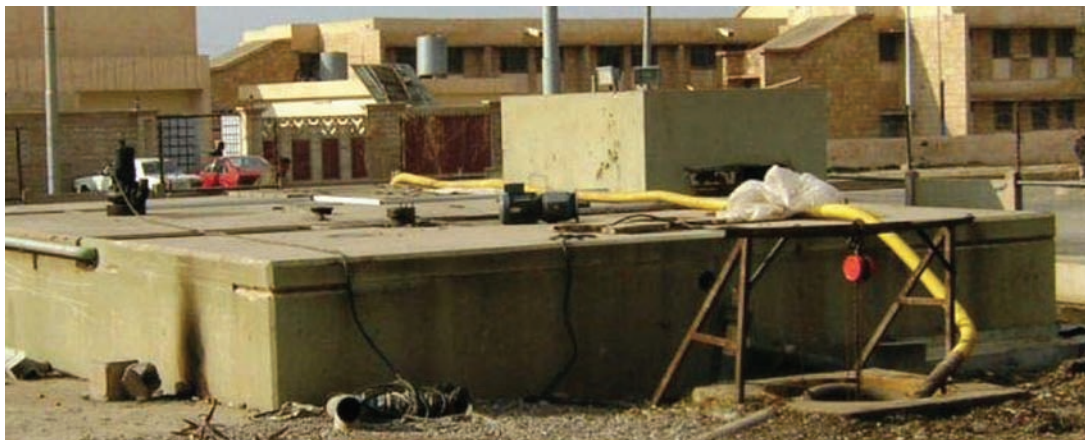
Before renovation, the septic tank was bypassed and hospital sewage was pumped from the cesspool to the municipal system. (USACE, January 4, 2005)
