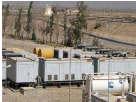
Seven Caterpillar generators. (Photo provided by USAID)
