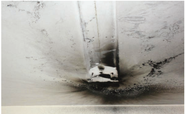
Unprotected high-voltage power cable wires exposed to leaking water.
