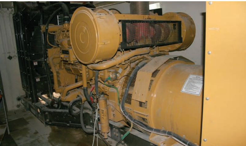
New generator used as a back up.
