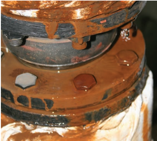
Evidence of water leakage from hot-water line.
