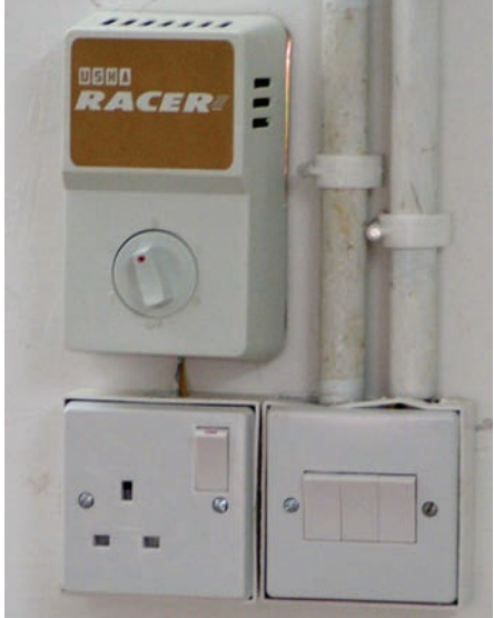
Wiring and components securely fastened to walls.
