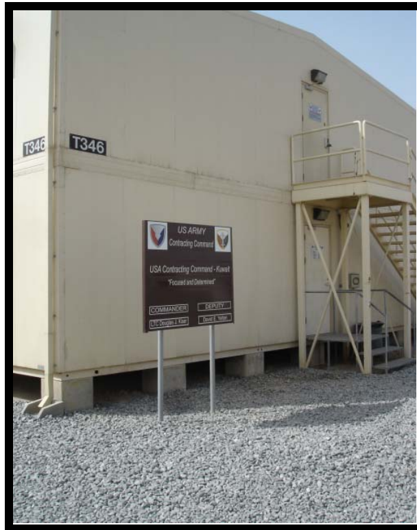
Figure 8. USACC-KU main building (T-346) 29
