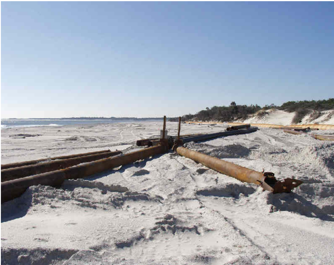
Figure 3. South Amelia Island O&M disposal area (January 25, 2001). Approximately 330,000 cubic yards of beach quality sand were placed as part of this multi-agency initiative
