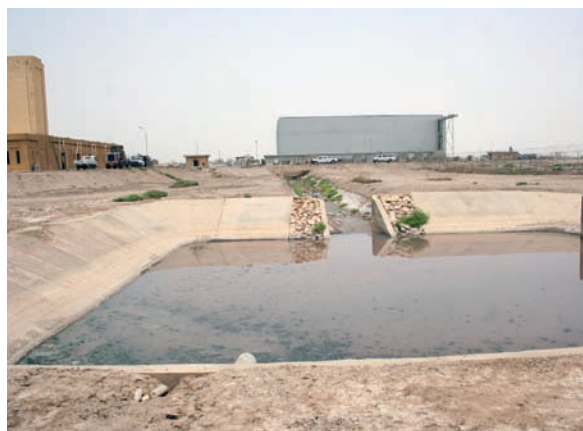
Storm drainage collection pond containing raw sewage.
