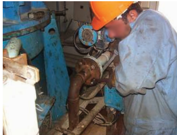
Rehabilitating pumps (picture courtesy of USACE).
