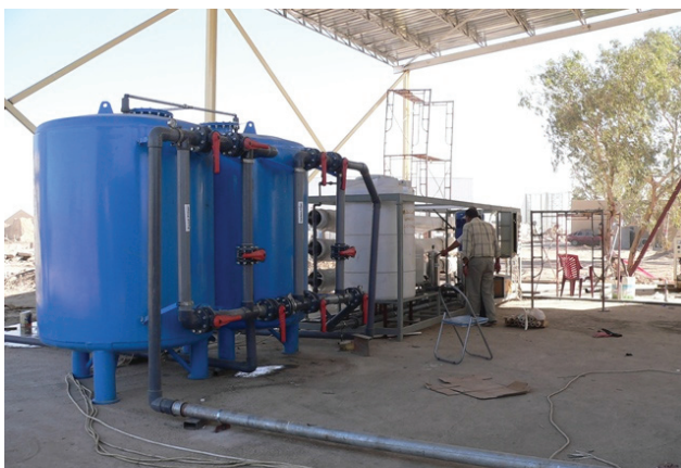
Reverse osmosis unit at installation (contractor-provided photo).
