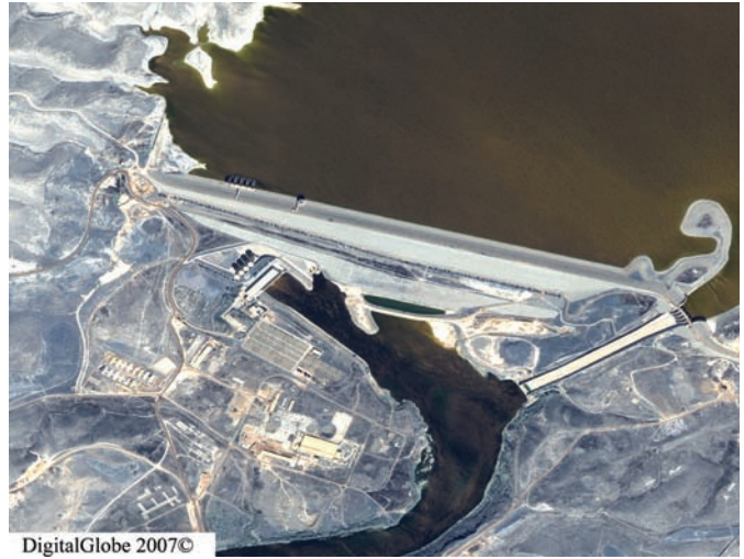
Aerial Image 4. Overview of the Mosul Dam, which SIGIR inspectors visited this quarter.
