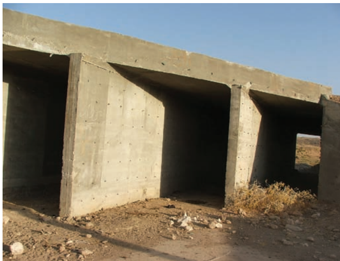
Site Photo 11. Box culverts for new road.
