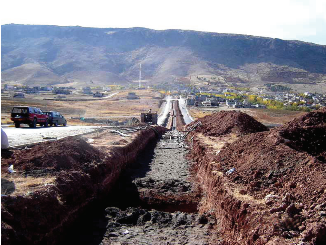
CERP-funded road construction.
