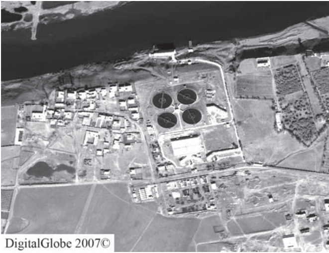
Aerial Image 3. Imagery overview of the Right Bank Drinking Water Treatment Plant taken on February 27, 2007.
