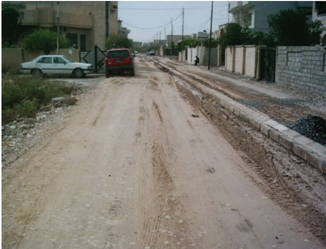
Site Photo 12. Road excavation, leveling, and rolling of the sub-grade (photo courtesy of USACE).
