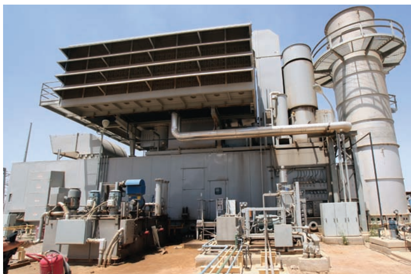
Site Photo 9. General Electric LM-6000 turbine unit.
