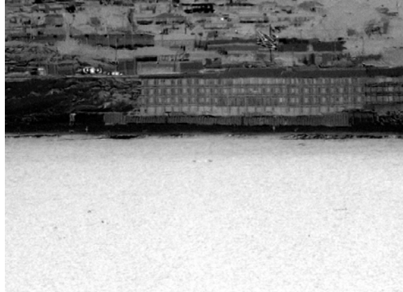
DOLP image of a hotel across the bay of Monterey Bay, CA on 8 August 2008 1342
