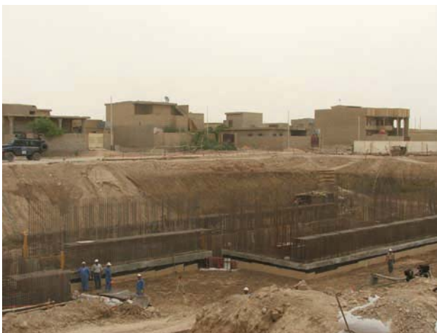
Falluja wastewater project: effluent pump station construction.
