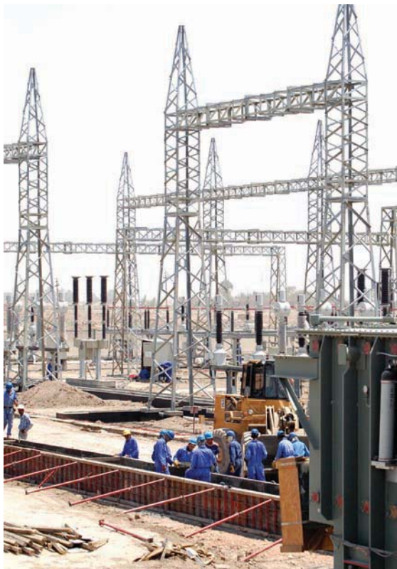
Construction of the Diwaniyah 132kV AIS Substation in Qadissiya now completed. (USACE photo)
