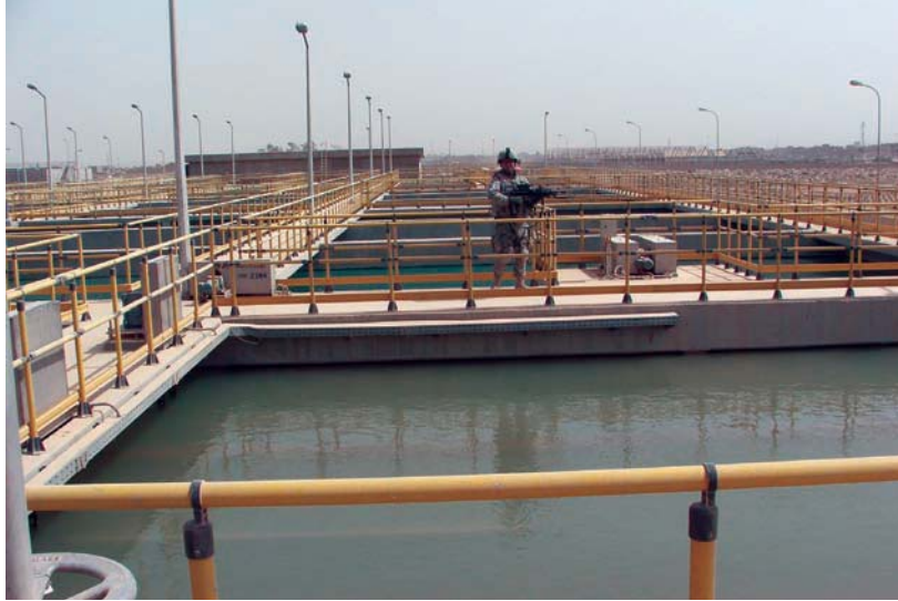
Sadr City water project: flocculation tanks.
