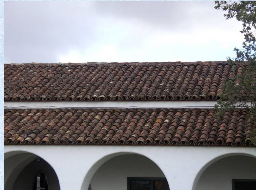
Tile roof with steep slope
