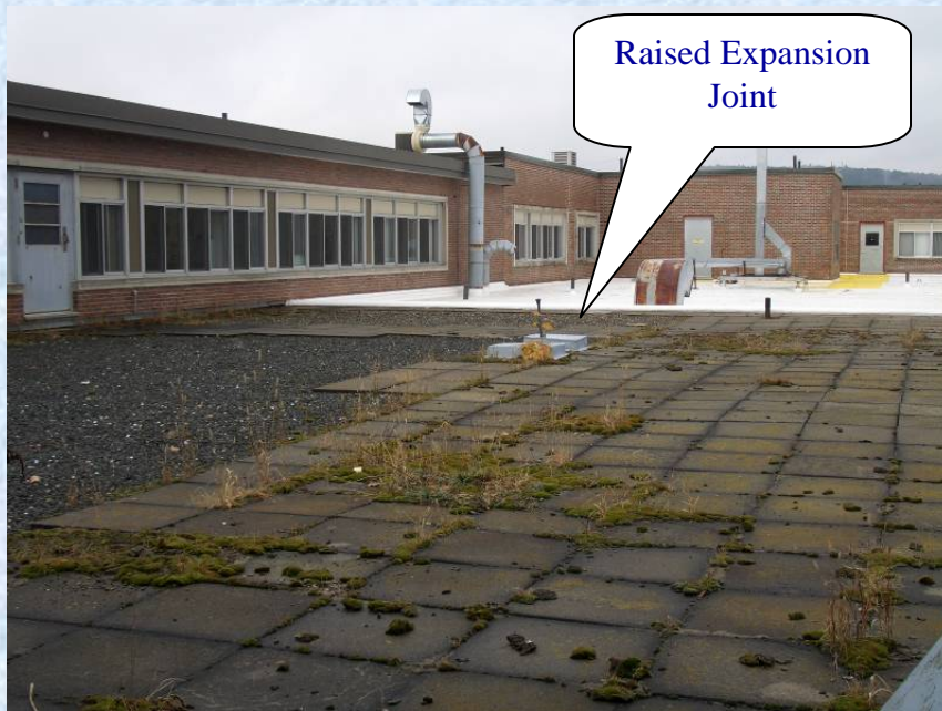
Built-up roof with three different surfaces
