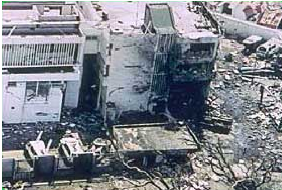
Figure 5 191 : Damage to the U.S. Embassy in Tanzania
