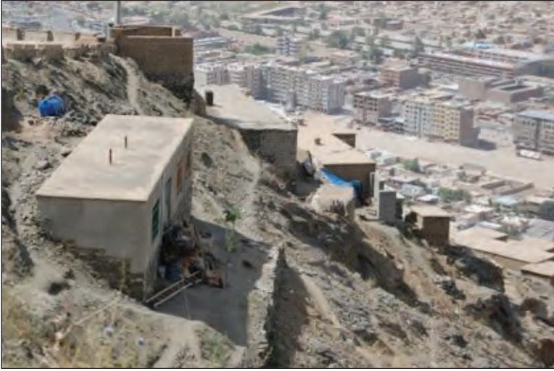
Figure 12. Informal Dwellings Built on Kabul Hillside. Source: Dr. Gregory Maassen, EMG.
