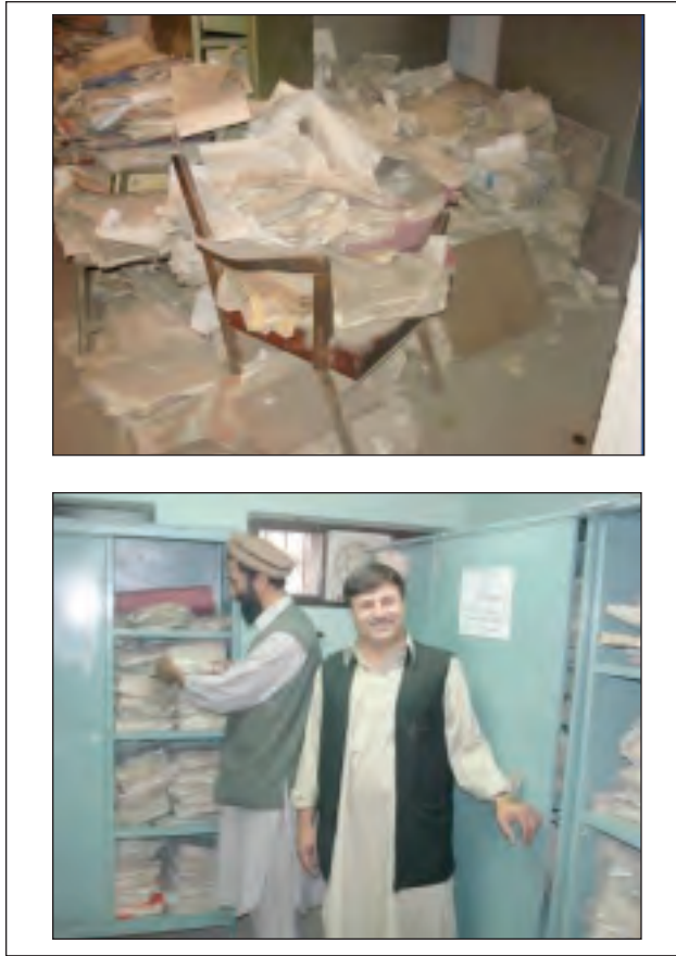
Figure 43. Mahkzan Rehabilitation Photos: Before and After. Source: LTERA.
