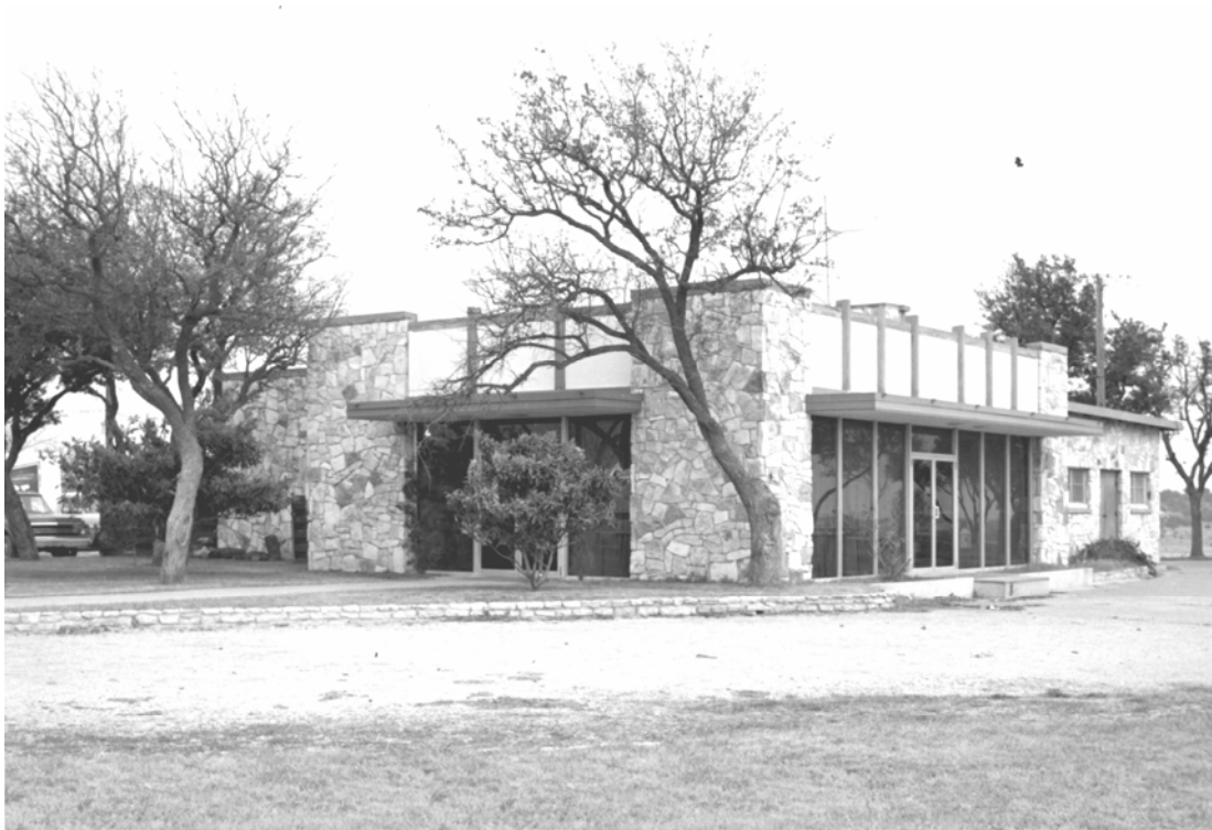
Figure 32. View of the Fort Hood Rod and Gun Club (NARA).
