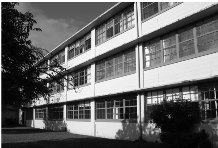
Figure 193. Original windows on H-Style barracks at Fort Lewis, WA (ERDC-CERL, 2004).
