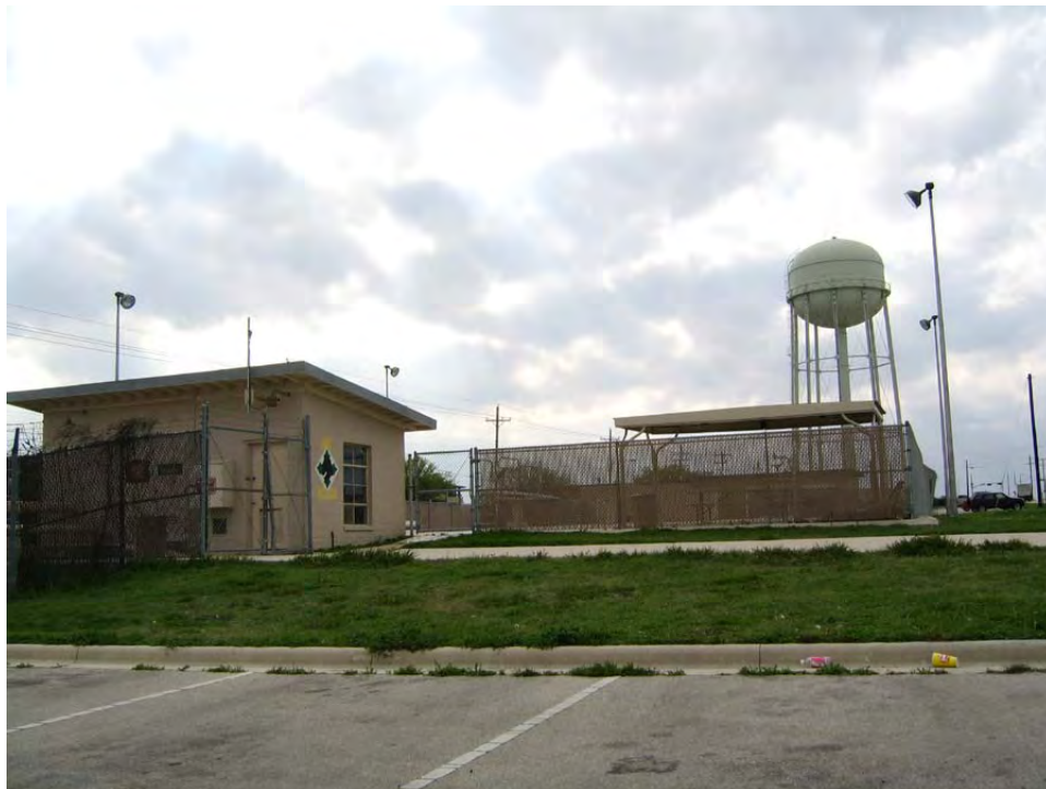
Figure 114: Photograph of swimming pool (Building 1676) located between Old Ironsides Ave and Hell on Wheels Avenue (ERDC-CERL 2004).
