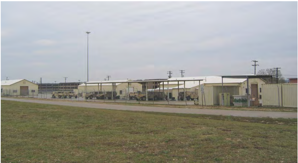
Figure 171: Motor pool for Killeen Base "A" Area (ERDC-CERL, 2004).
