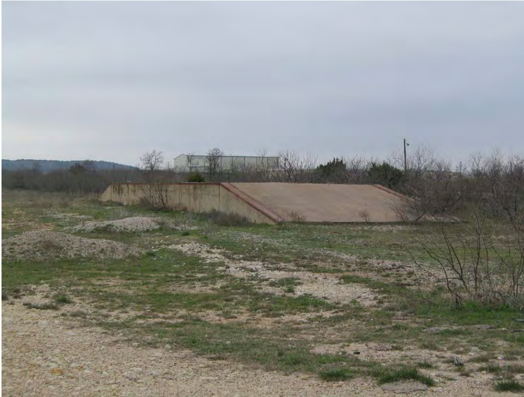
Figure 123: Railroad loading ramps at North Fort Hood (ERDC-CERL, 2004).
