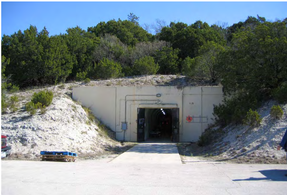
Figure 160: Entrance to converted “A” structure #92107 (ERDC-CERL, 2004).
