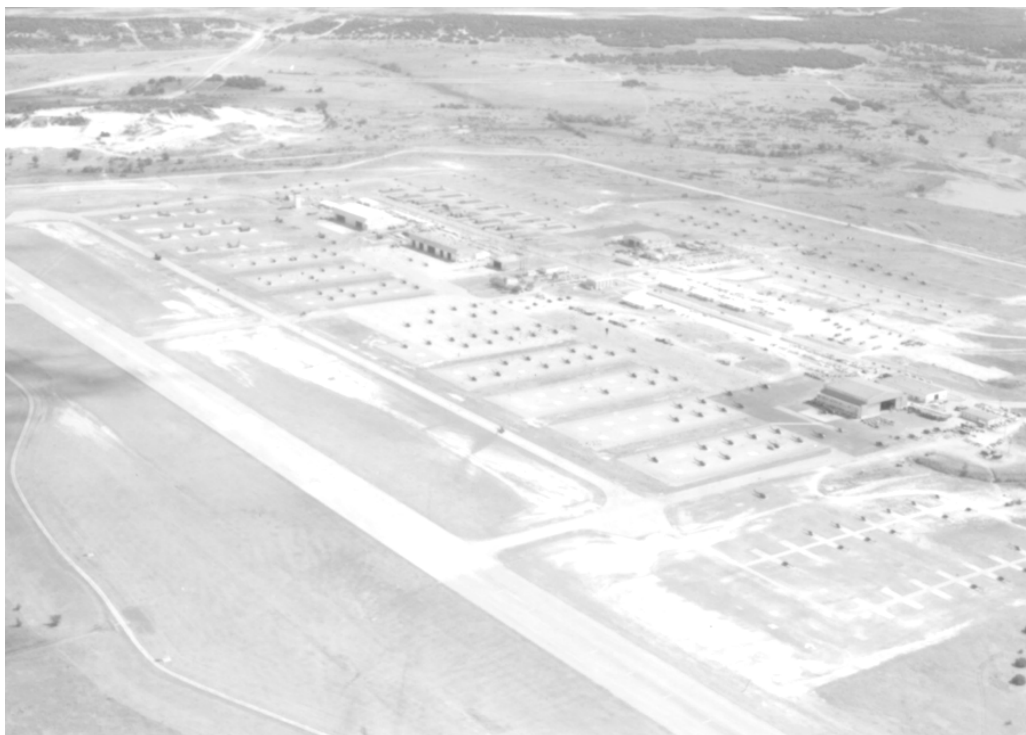
Figure 60: Aerial view of Hood Army Airfield, circa August 1977 (NARA).
