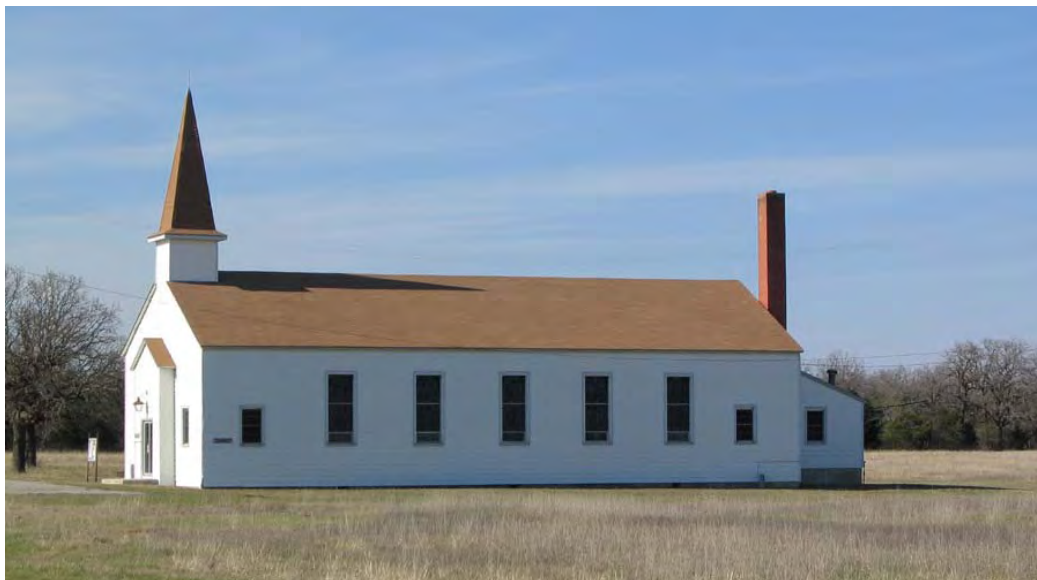
Figure 129: WWII era church at North Fort Hood (ERDC-CERL, 2004).
