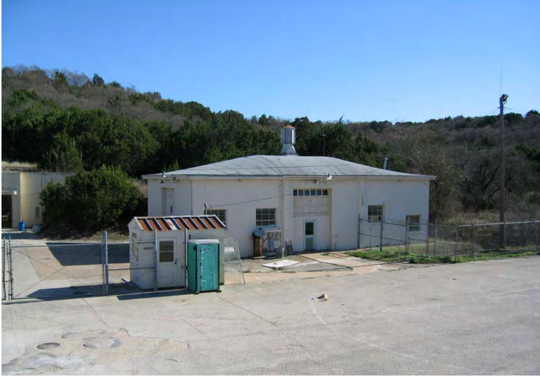
Figure 157: Battery charging building #92045 associated with Plant #92050 (ERDC-CERL, 2004).
