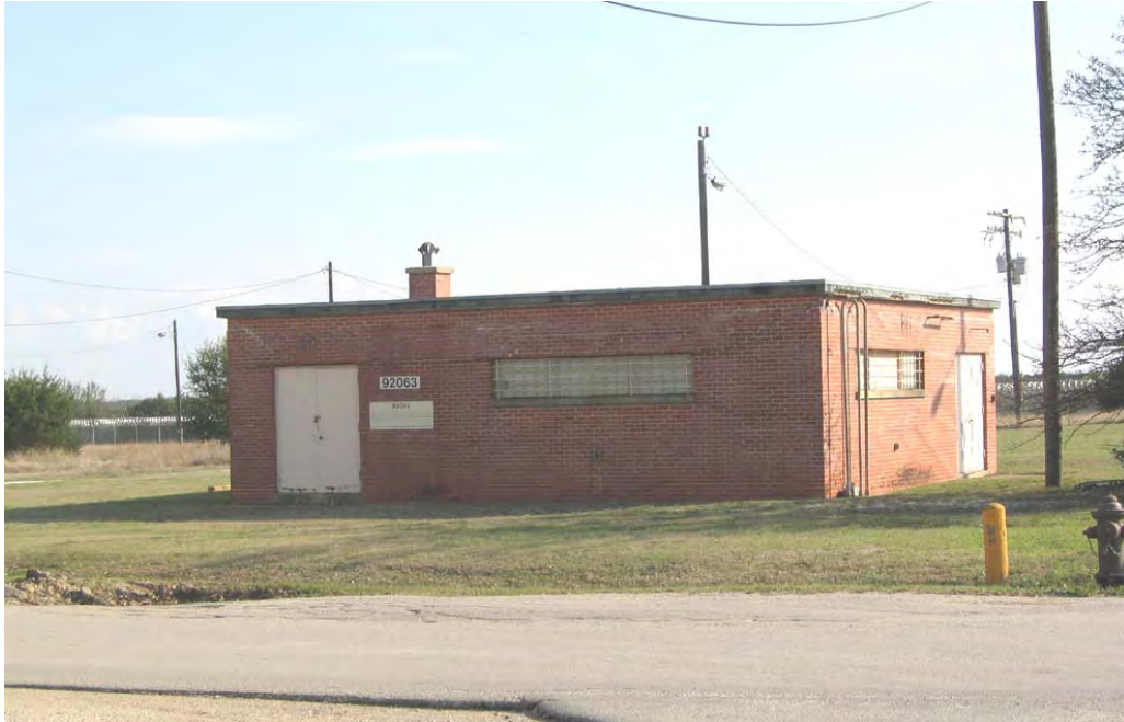
Figure 163: Radio reception building #92063 (ERDC-CERL, 2004).
