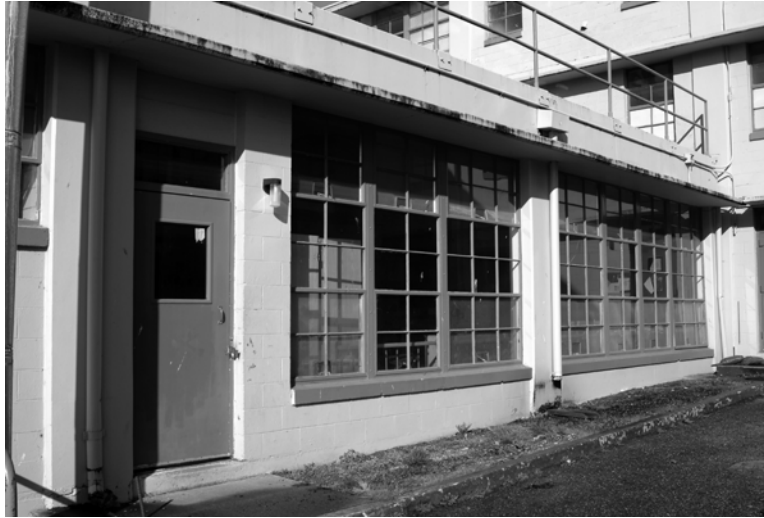
Figure 194. Original mess hall windows on H-Style barracks at Fort Lewis, WA (ERDC-CERL, 2004).
