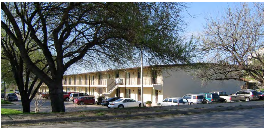
Figure 92: Photograph of Paxon House along Hood Road (ERDC-CERL 2004).
