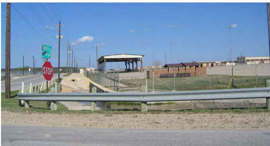
Figure 96: Photograph of wash area and wastewater runoff system in motor pools (ERDC-CERL 2004).
