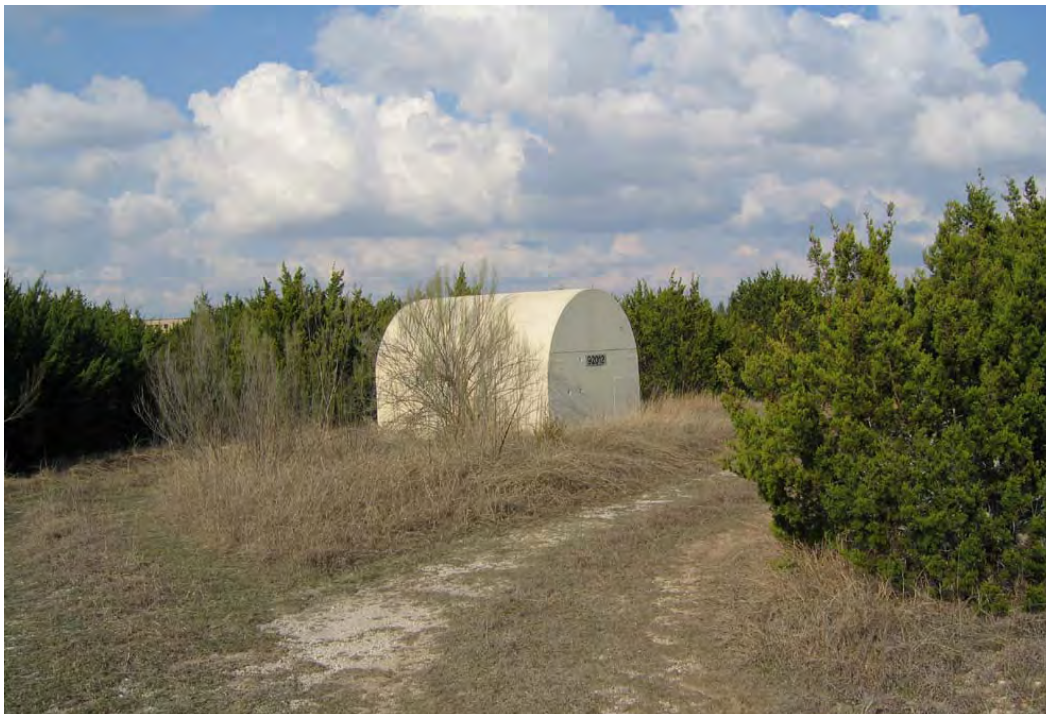
Figure 162: Small arms ammunition storage building #92012 (ERDC-CERL, 2004).
