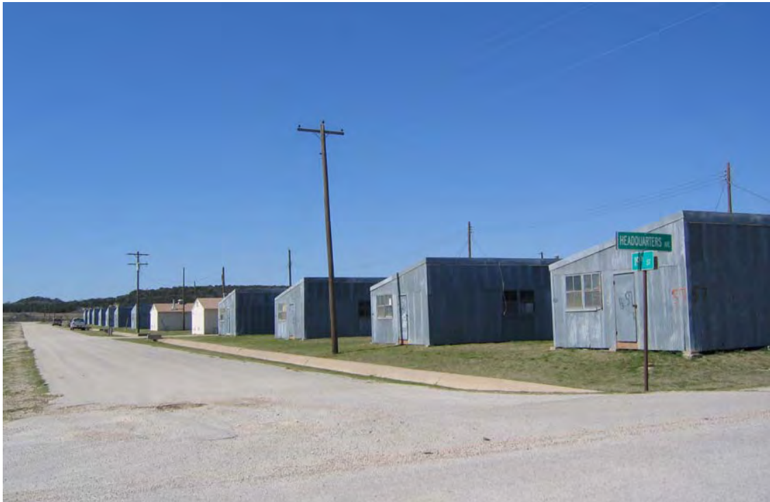
Figure 135: Photograph of metal temporary hutments along 19th Street (ERDC-CERL, 2004).
