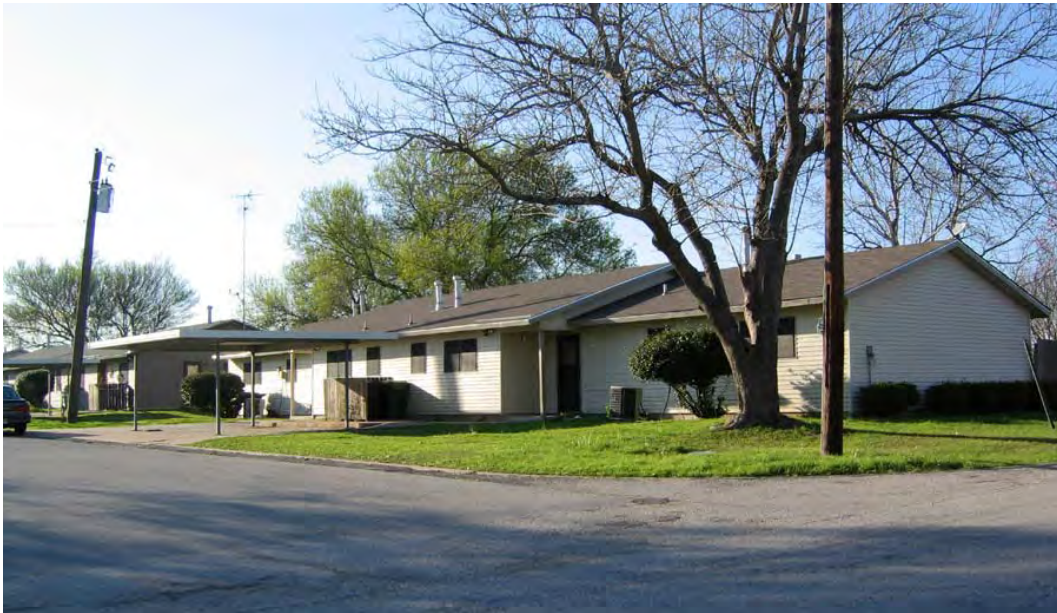
Figure 82: Photograph of Venable Village at Fort Hood (ERDC-CERL 2004).
