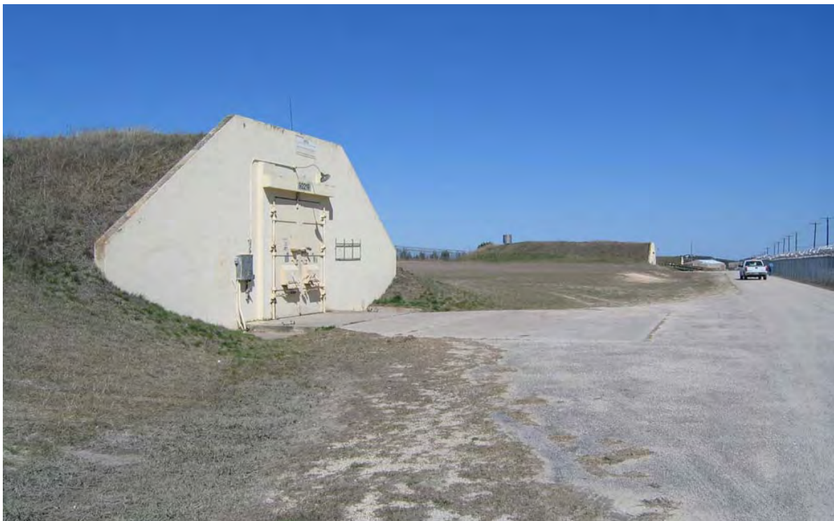
Figure 159: Above-ground igloo #92219 along North Road (ERDC-CERL, 2004).
