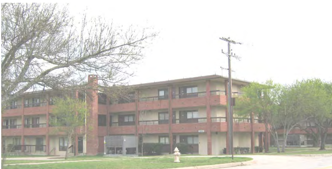
Figure 72: Rolling pin barracks (Building 12004) at Fort Hood (ERDC-CERL 2004).
