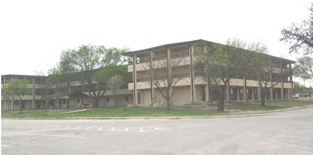
Figure 70: H style barracks (Building 14020) at Fort Hood (ERDC-CERL 2004).
