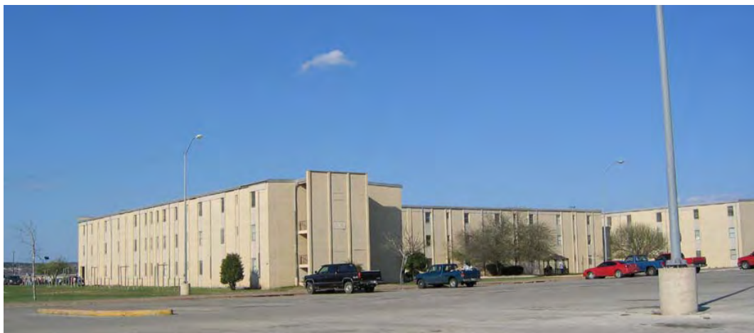
Figure 74: A-style barracks (Building 31007) at Fort Hood (ERDC-CERL 2004).
