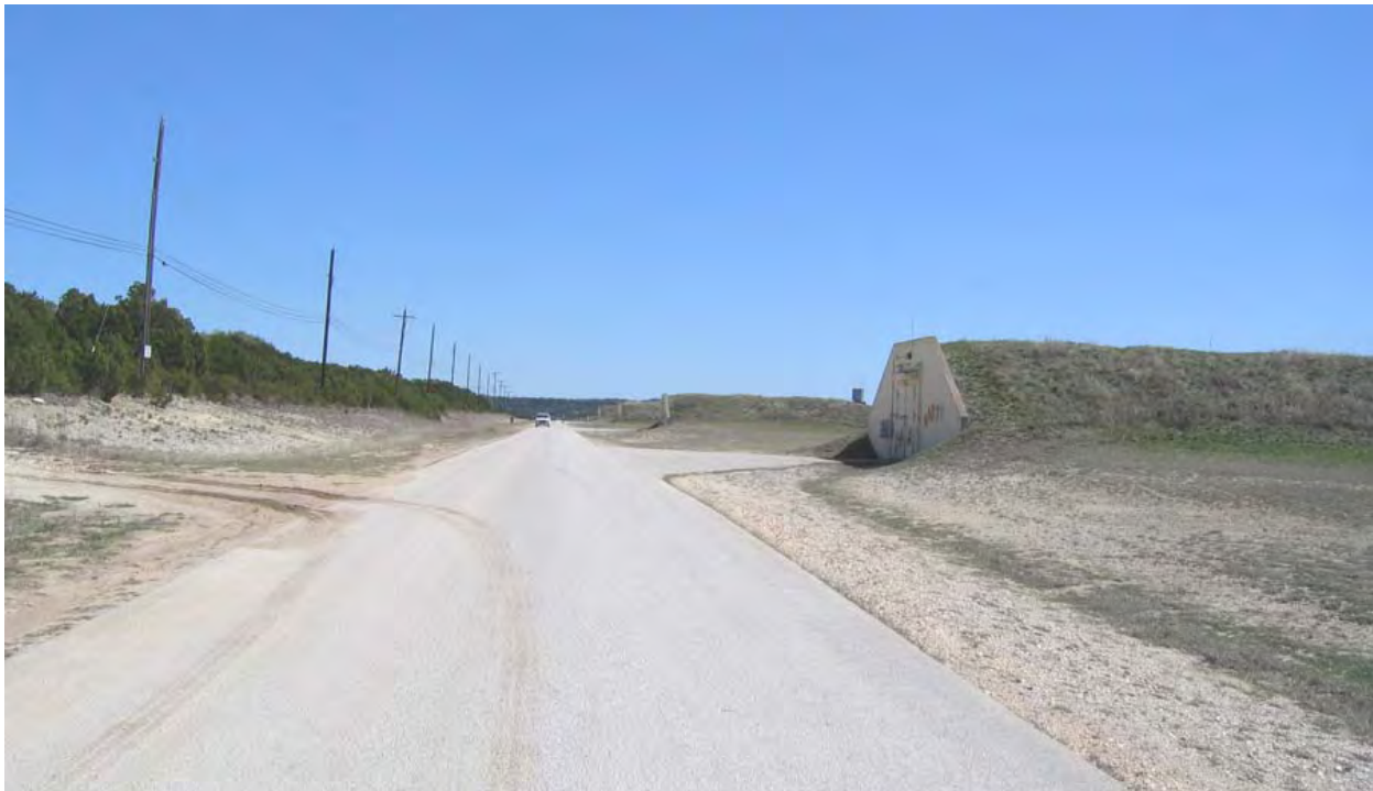
Figure 151: Row of above-ground igloos along South Road (ERDC-CERL, 2004).
