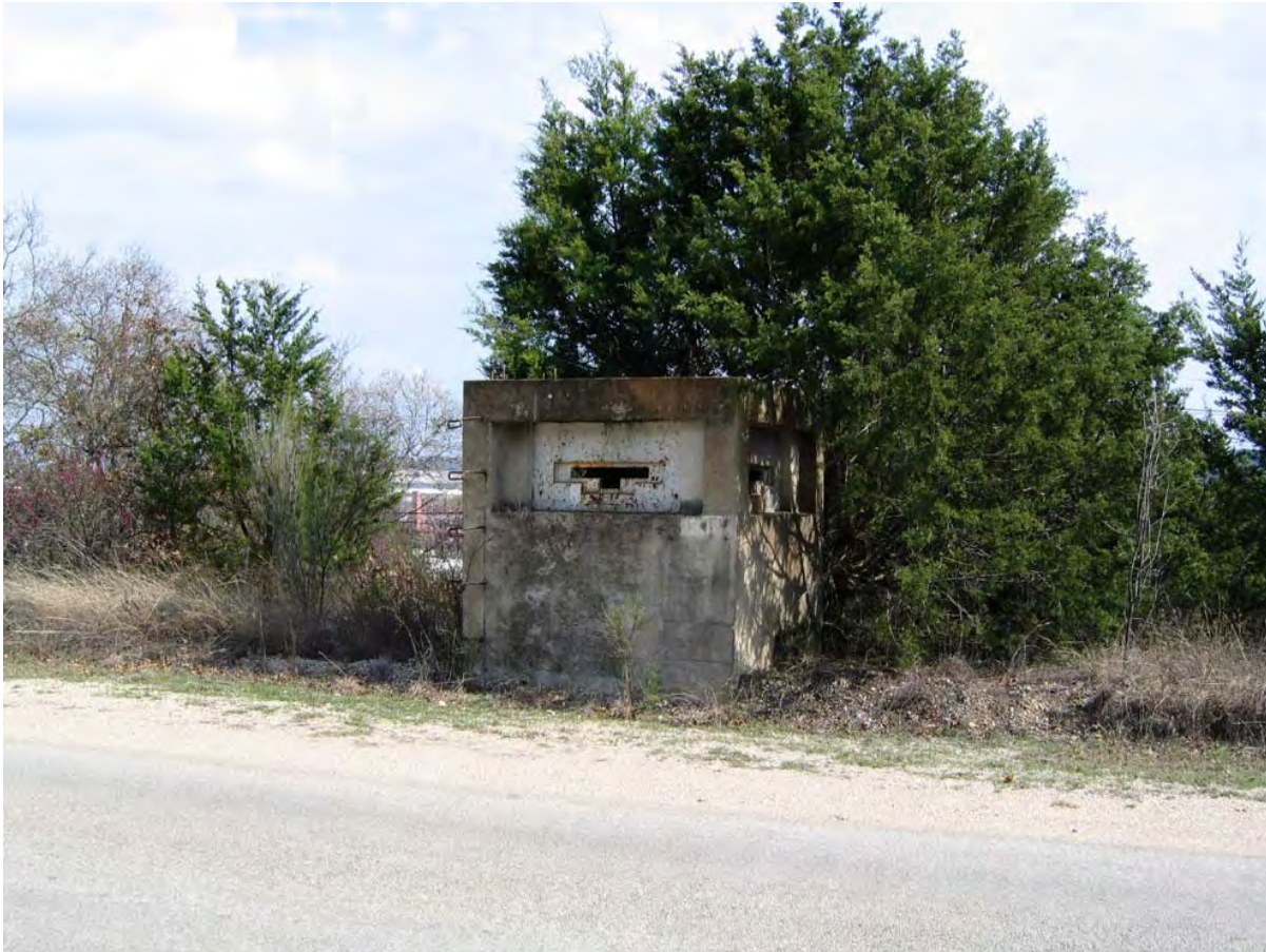
Figure 154: Vegetation obstructing views from pillbox (ERDC-CERL, 2004).
