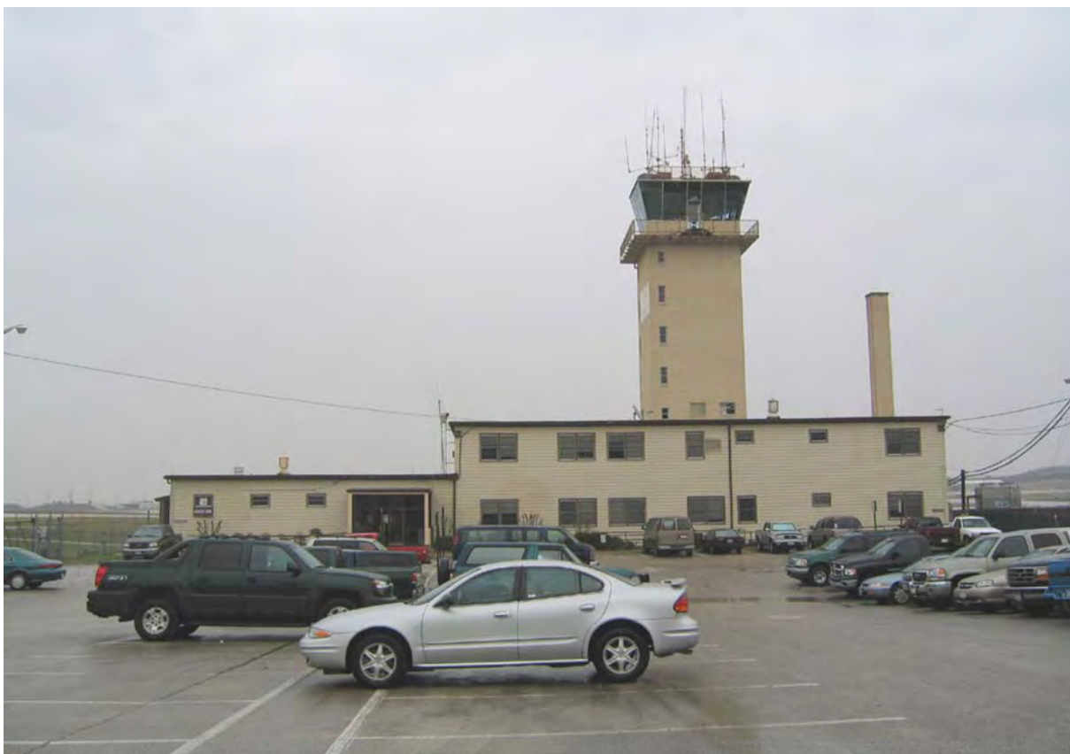
Figure 172: Former flight control tower and snack bar #90049 (ERDC-CERL, 2004).
