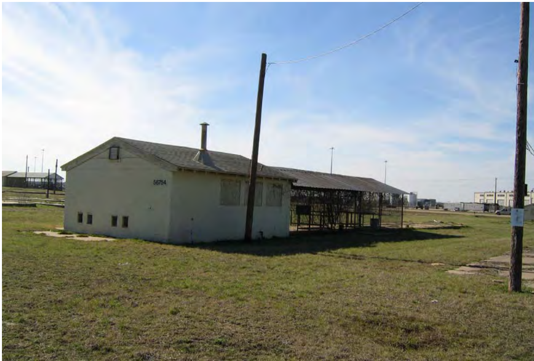
Figure 132: Dining Facility #56754 built in 1951 (ERDC-CERL, 2004).
