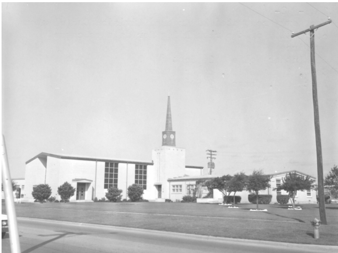
Figure 31. Newly rebuilt 2 nd AD Chapel (NARA).
