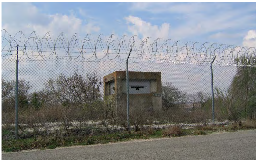
Figure 164: Pillbox #92037 and new non-compatible fencing (ERDC-CERL, 2004).
