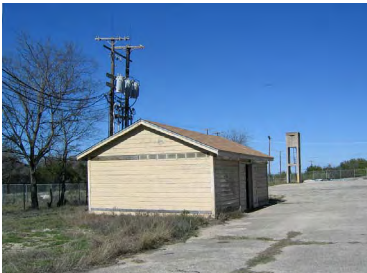
Figure 156: Structures including bldg 92043 and tower, associated with plant #92050 (ERDC-CERL, 2004).
