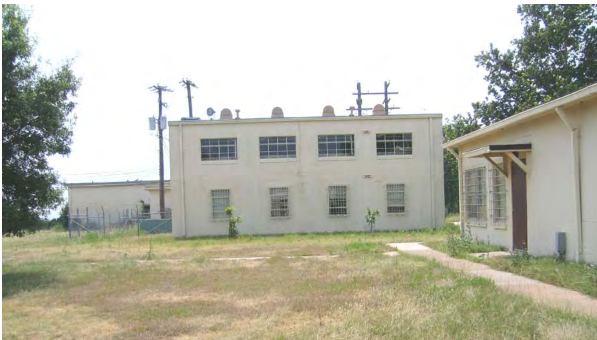
Figure 179: Cluster of buildings (#90064-6) at Radar Hill (ERDC-CERL, 2005).
