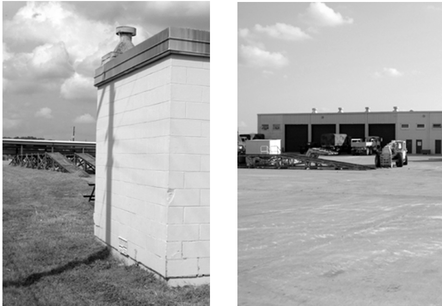
Figure 186. Grease racks shown in various locations within select motor pools (Stupich).
