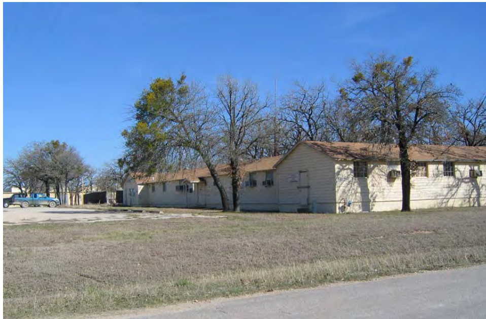
Figure 131: WWII era administration building #56327 (ERDC-CERL, 2004).
