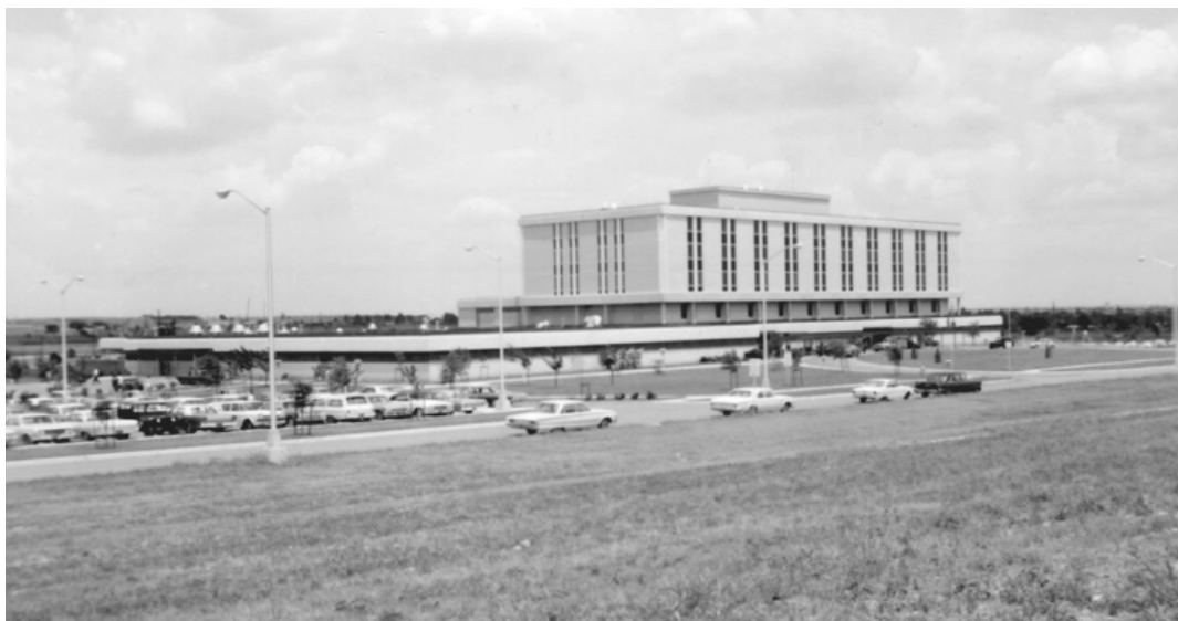
Figure 89: Front ground level view of Darnall Army Hospital from southwest corner, July 1966 (NARA).
