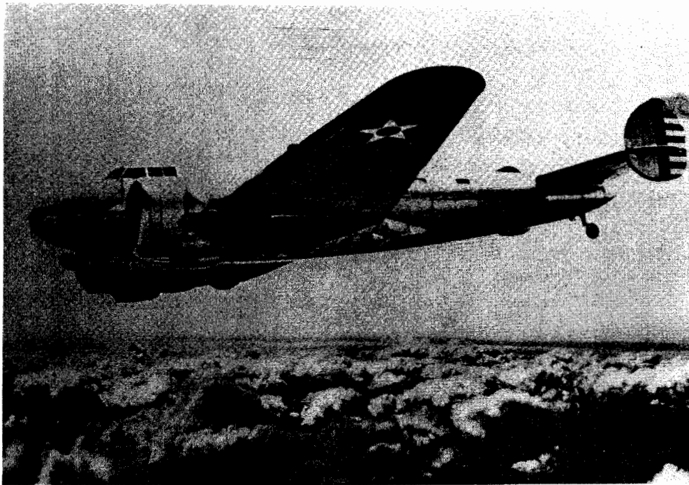
Fig I-4 XC-35, first successful pressurized sealed cabin aircraft. Armstrong specified the physiological requirements for the cabin atmosphere. The cabin pressurization system was manually controlled by Armstrong or Pvt. Whitney on each test flight.
