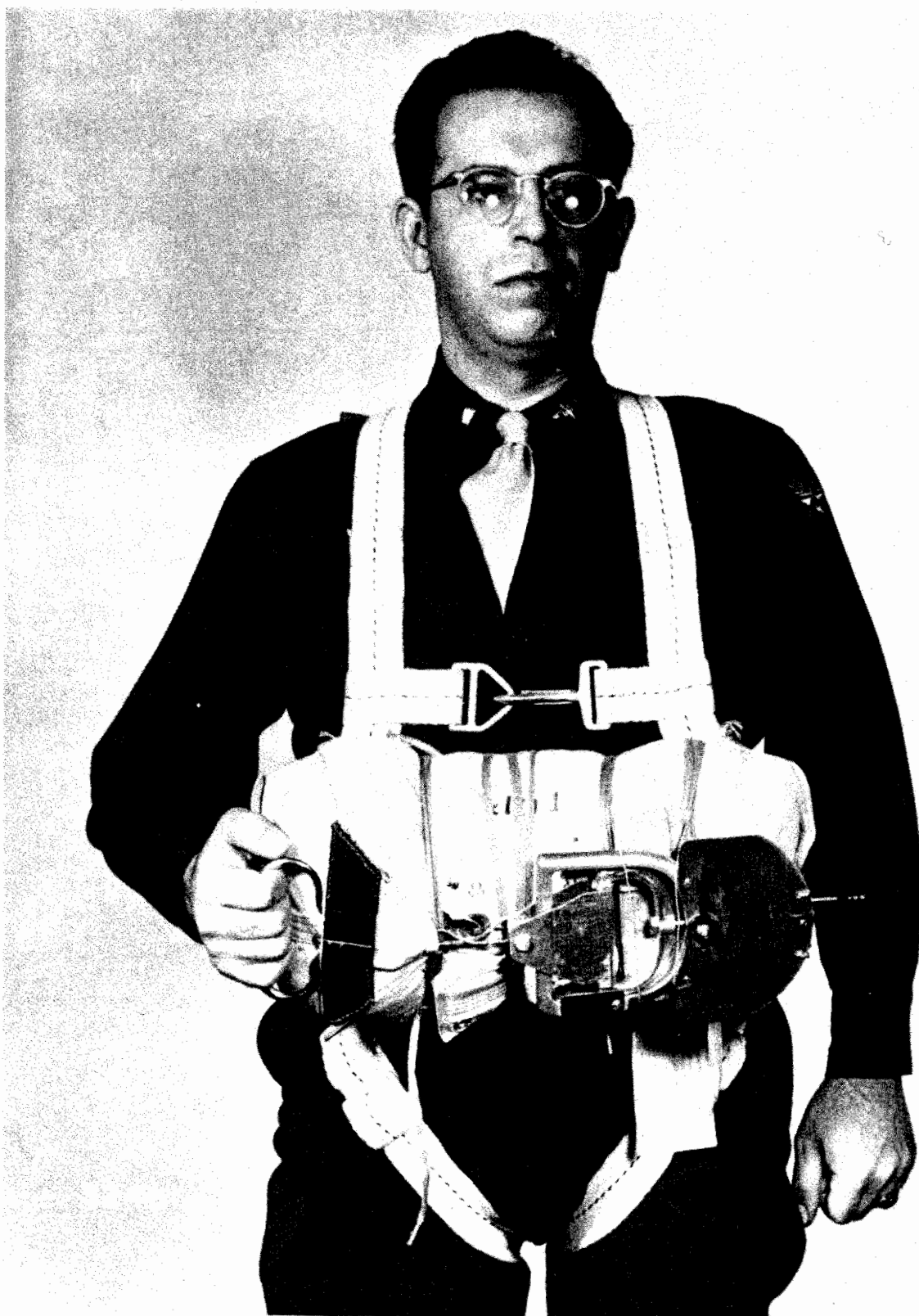
Fig II-18 High altitude free fall parachute program. Lt. Martin demonstrating parachute pull force test unit 1943.
